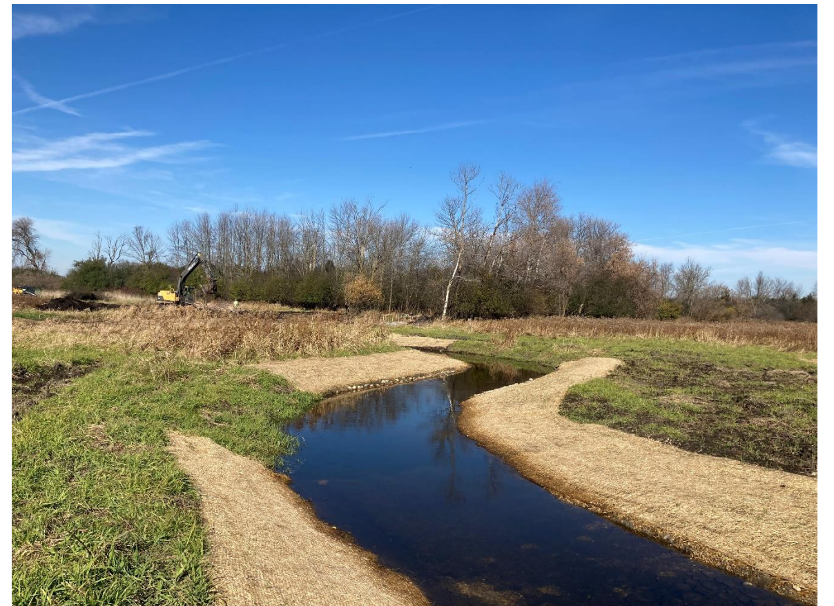
TPC Mason Creek stream and wetland restoration, Waukesha Co.
