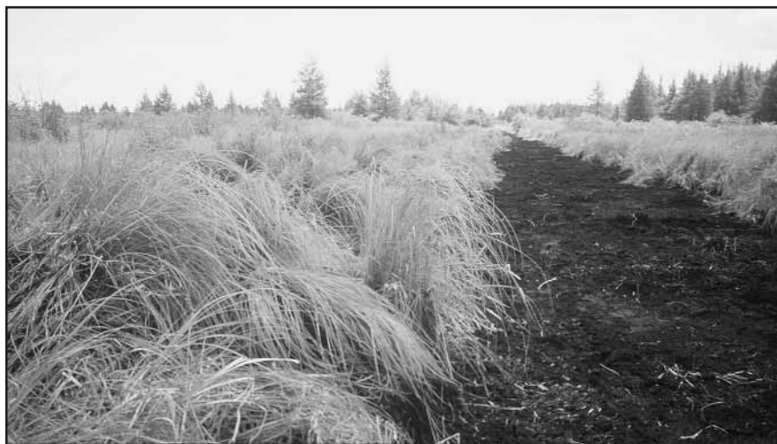
Ditch at Summerton Bog with original spoil bank that was on the right now in ditch and native sedges placed on top of ditch fill.
