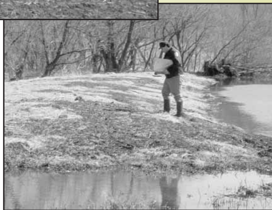
Seeding of dike to immediately stabilize fresh soil surfaces.
