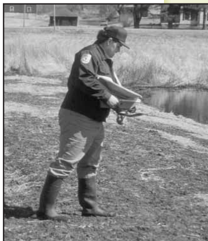
Seeding of dike to immediately stabilize fresh soil surfaces.
