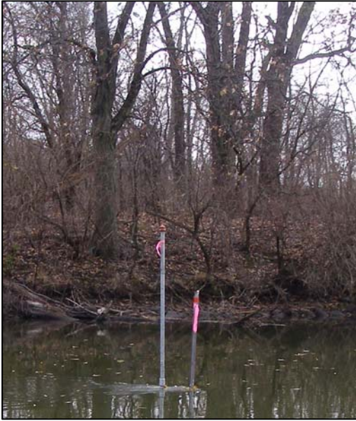
Photo 4 - Example of a lakebed piezometer nest. While a single temporary piezometer will typically be installed, multiple piezometers may be used to evaluate vertical gradients beneath the lakebed.
