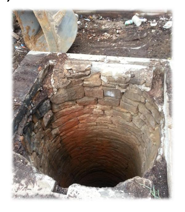
• Pit: Below ground structure that may contain the well, pump, pressure tank, valves, etc.
