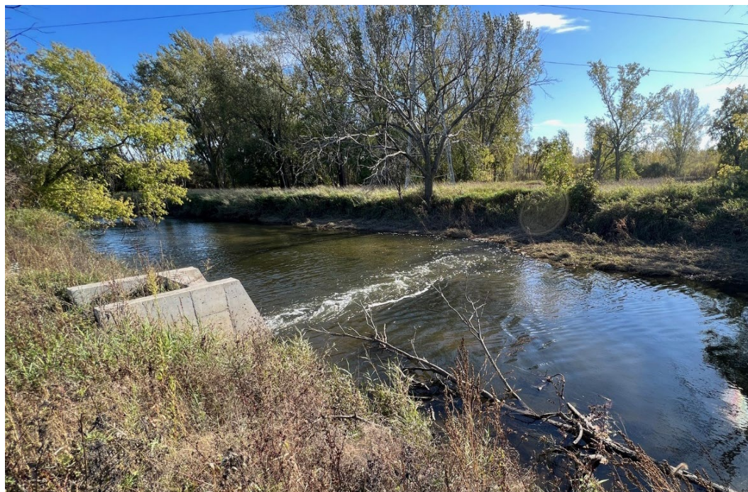
Figure 6-9. Return Flow Outfall Structure at the Root River
