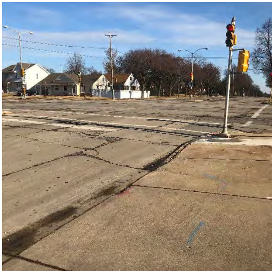
Photo 1 Looking east at the intersection of Howard Avenue and 60th Street
