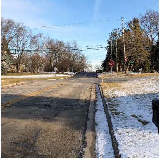
Photo 70 Looking east at the intersection of Observatory Road and Calhoun Road
