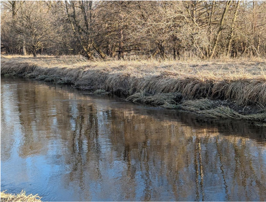
Image 3.3 – Bank on top, undercut with slumped material, covered with grass.
