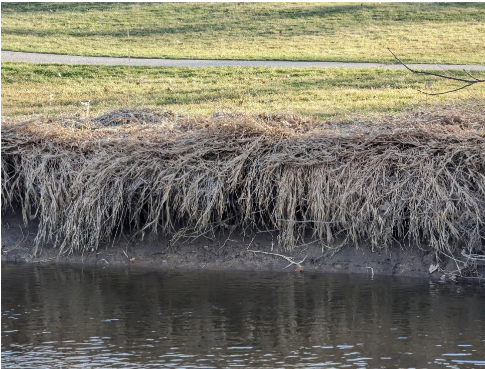
Image 2.2 – Bank, undercut, somewhat hidden due to overhanging grass.
