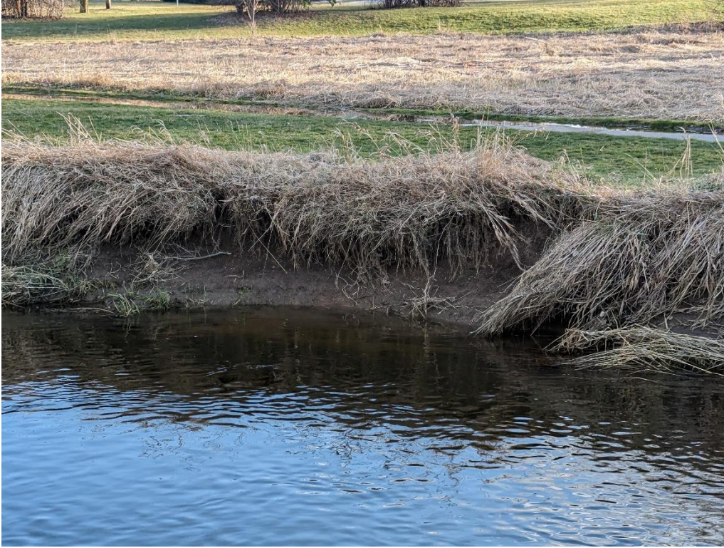
Image 1.2 – Bank undercut, covered with grass
