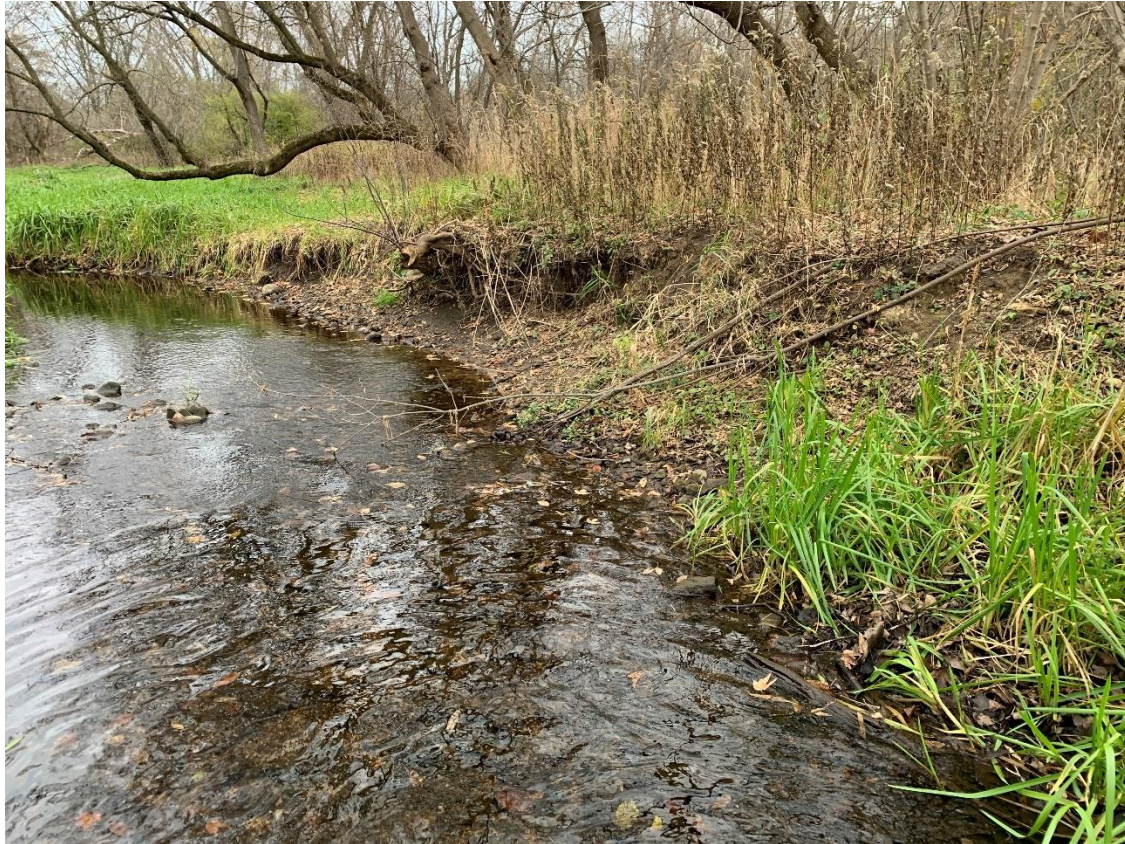
Image 1.1 – Bank on right, undercut with slumped sections in stream, covered with grass
