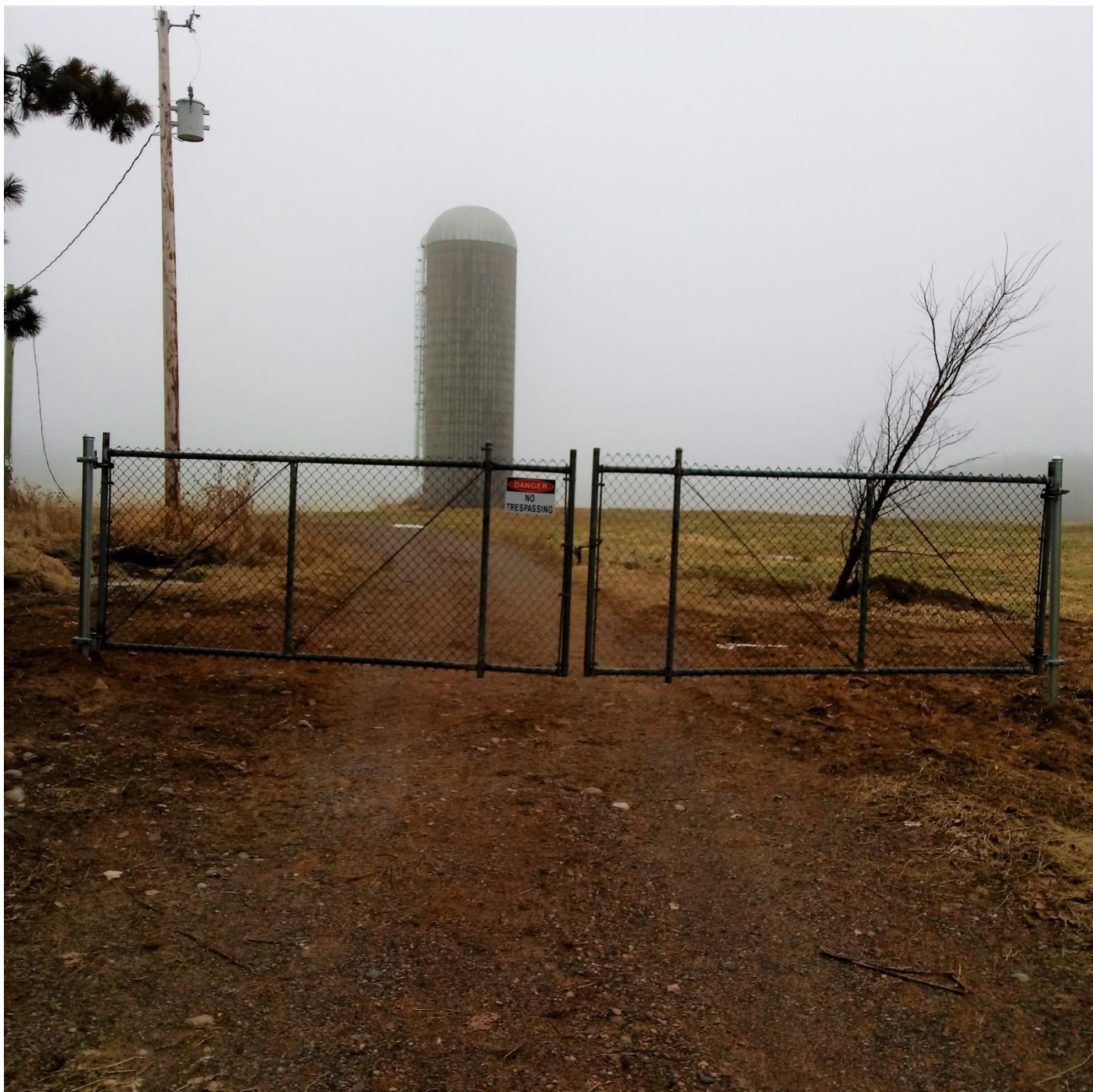
Newly installed gate at the Hawkins WQT site.
