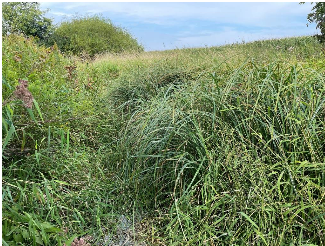
Photo 4. Clayton Br. Near outfall confluence looking downstream.
