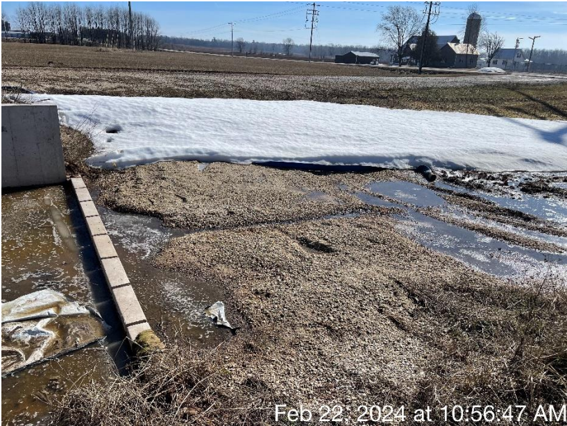
Photo 24. The concrete and gravel spreader bar that is designed to disperse runoff across the VTA. Concentrated flow was present at the time of the inspection.
