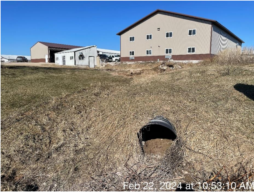
Photo 36. The inlet associated with the outlet pictured in Photo 35. The culvert accepts runoff from the driveway area west of the feed storage area. This photo was taken facing south.
