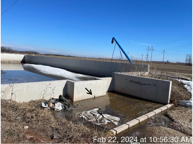
Photo 24. The concrete and gravel spreader bar that is designed to disperse runoff across the VTA. Concentrated flow was present at the time of the inspection.
