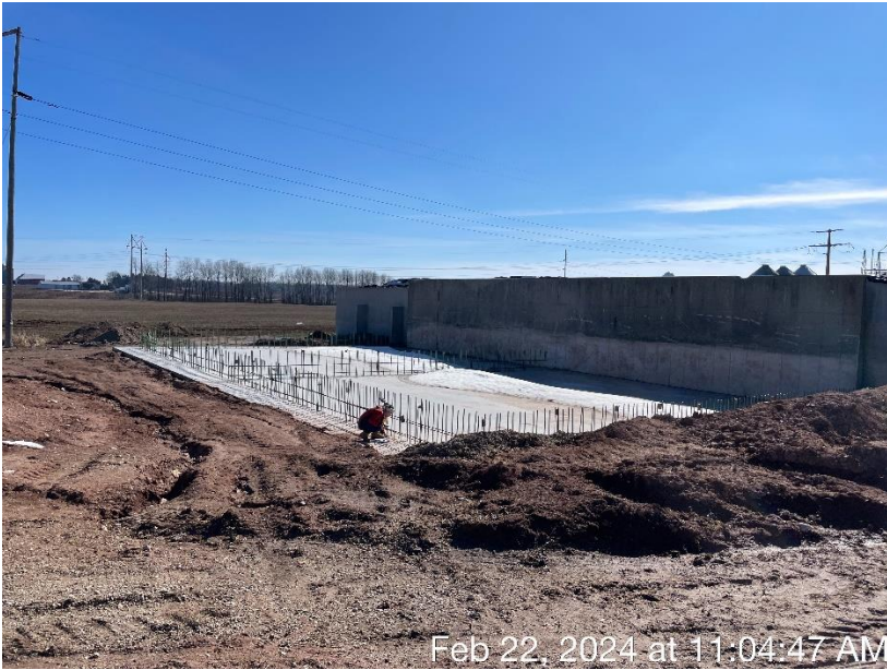
Photo 20. The flow path of runoff towards the collection basin, located on the east side of the feed storage area.
