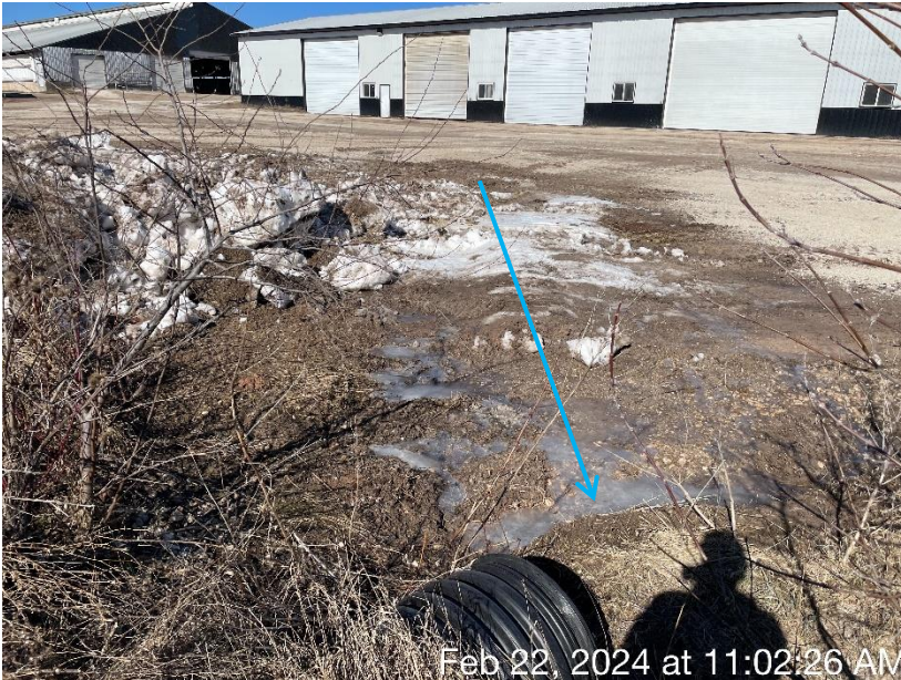
Photo 37. The flow path of stormwater towards the culvert pictured in Photo 36.
