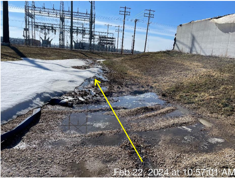
Photo 26. The VTA that handles runoff from the feed storage area. The yellow area arrow represents the flow path of runoff across the VTA.
