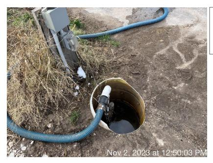
**Photo 35.** The interim runoff collection system for the feed storage area at Site 1. A 55-gallon drum and a sump pump transfers process wastewater to a manure tanker.
