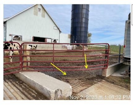
**Photo 9.** The concrete feedlot at Site 2. The yellow arrows represent the flow path of runoff on the lot.
