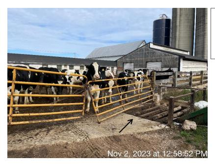
**Photo 4.** The runoff collection basin that accepts runoff from the concrete lot at Site 1. Manure is then augured from the basin directly into land application equipment.
