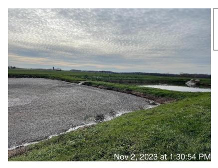
**Photo 22.** The earthen berm that separates WSF 1 and WSF 2 at the Milking Site. Manure flows through a concrete weir to WSF 2.
