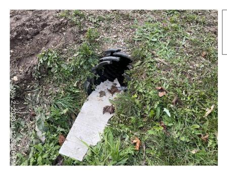
**Photo 51.** The inlet from the culvert located on the north side of the feed storage area. There was no evidence of runoff entering the culvert.
