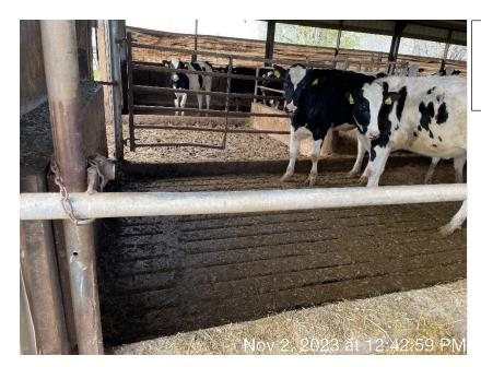
**Photo 19.** The floor drain that collects manure and process wastewater from the heifer barn at Site 1. Manure is manually pushed into the basin.
