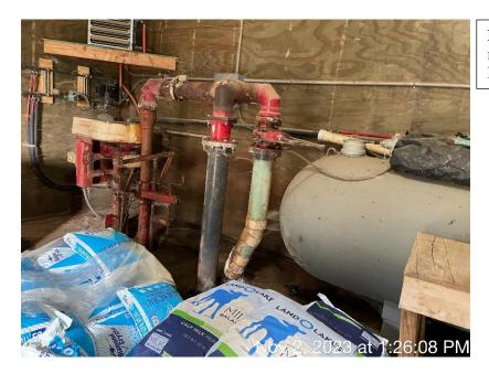
**Photo 31.** The transfer pump that sends manure from the reception tank in Photo 30 to WSF 1.
