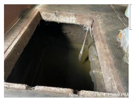
**Photo 30.** A concrete reception tank at the Milking Site that accepts manure from the freestall barn and conveys the manure to WSF 1.
