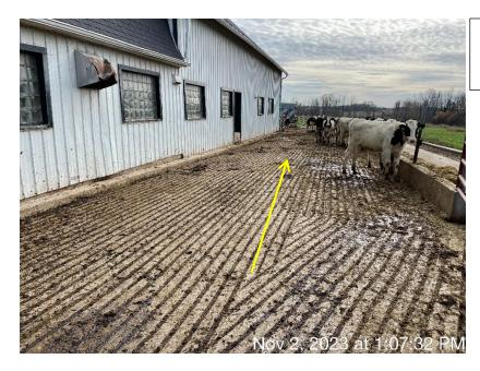
**Photo 7.** The outdoor concrete feedlot at Site 2. The yellow arrow represents the flow path of runoff on the barnyard.
