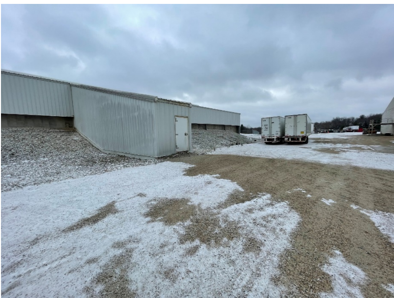
Photo 2: Building where manure enters the manure storage from the barns. Photo facing south.
