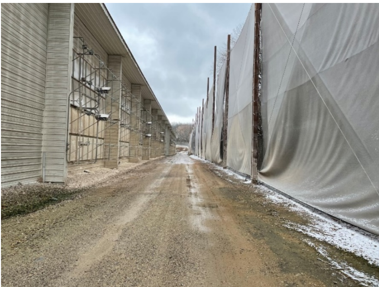
Photo 15: Area north of Barn 5. Traps are used to limit the dust leaving the production area. Photo facing west.
