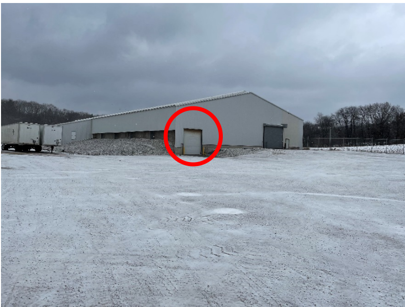
Photo 1: Manure storage building at S&R Egg LaGrange facing north. Loading area indicated with red circle.
