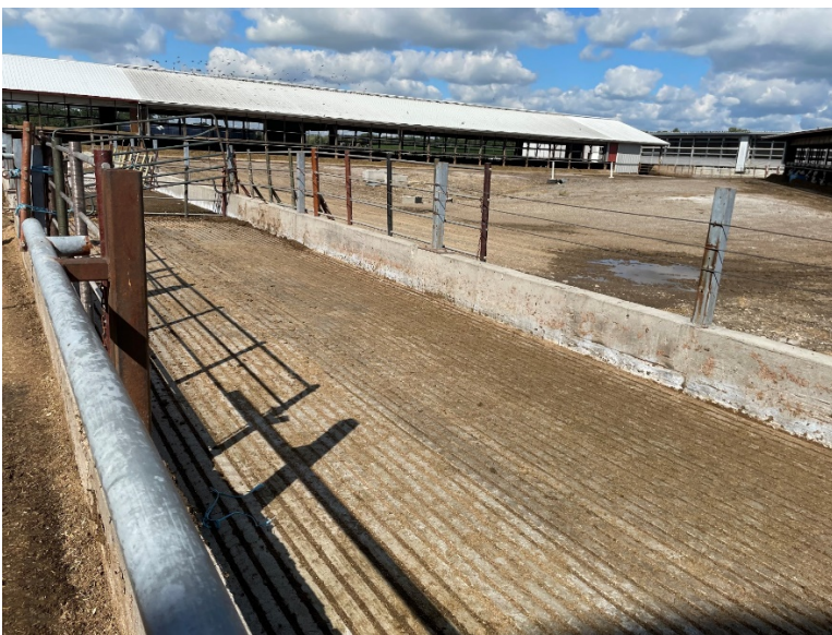
Photo 6: Cattle lane outside of the big heifer barn facing west.
