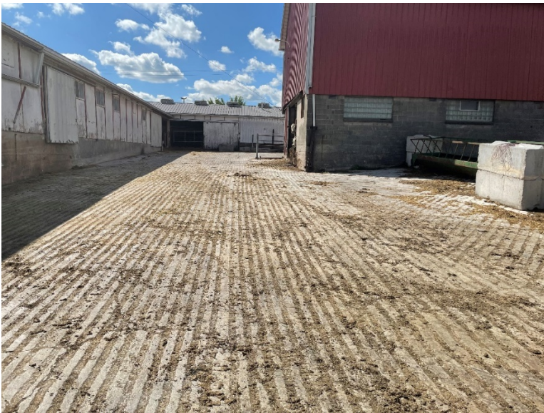
Photo 5: Cattle lane outside of the special needs barn facing south.
