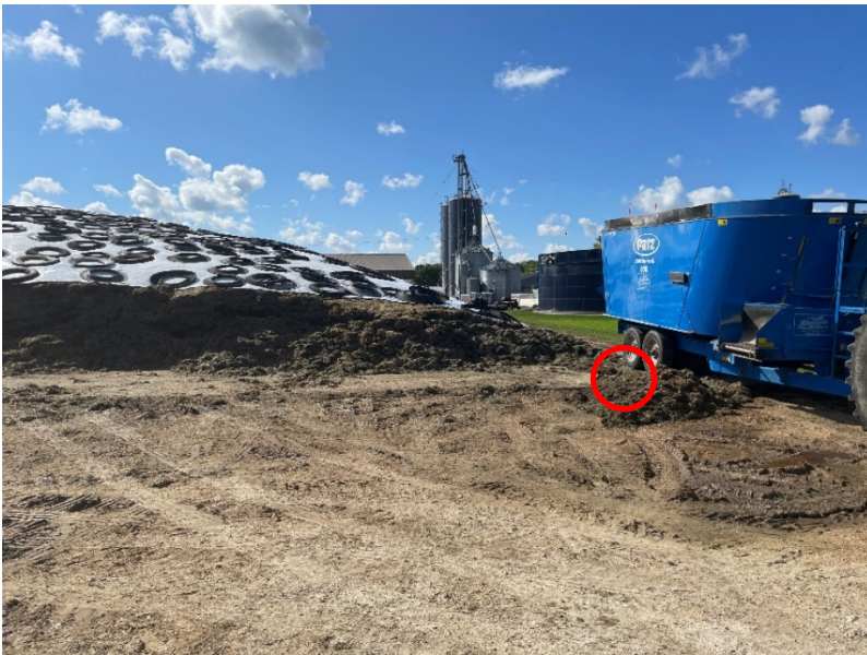
Photo 21: North side of FSA 2 facing south. Red circle indicates location of future runoff controls.
