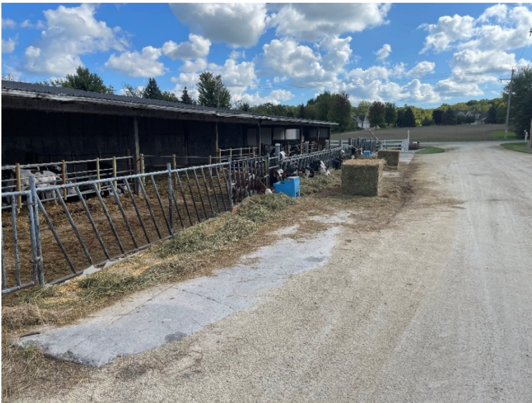
Photo 2: South side of the outdoor lot facing east.
