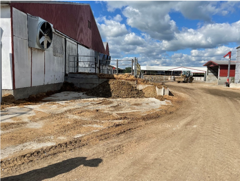
Photo 16: Separated solids to be placed for bedding outside barn facing west.
