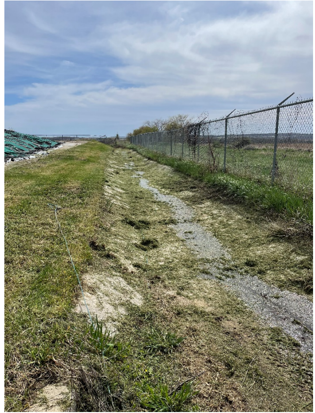
Photo 8 - Feed storage area runoff control conveyance. Photo taken facing east.
