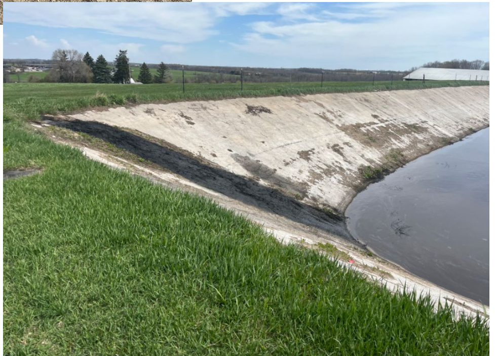
Photo 4 (right)- WSF3, black on side wall where petroleum product was placed. Photo taken facing northeast.
