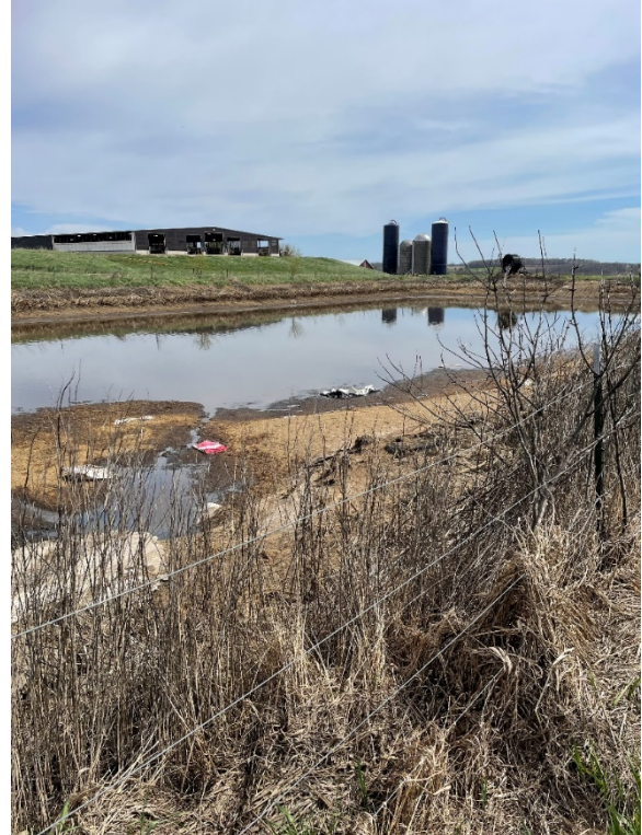
Photo 10- Feed storage area runoff control basin. Photo taken facing northeast.
