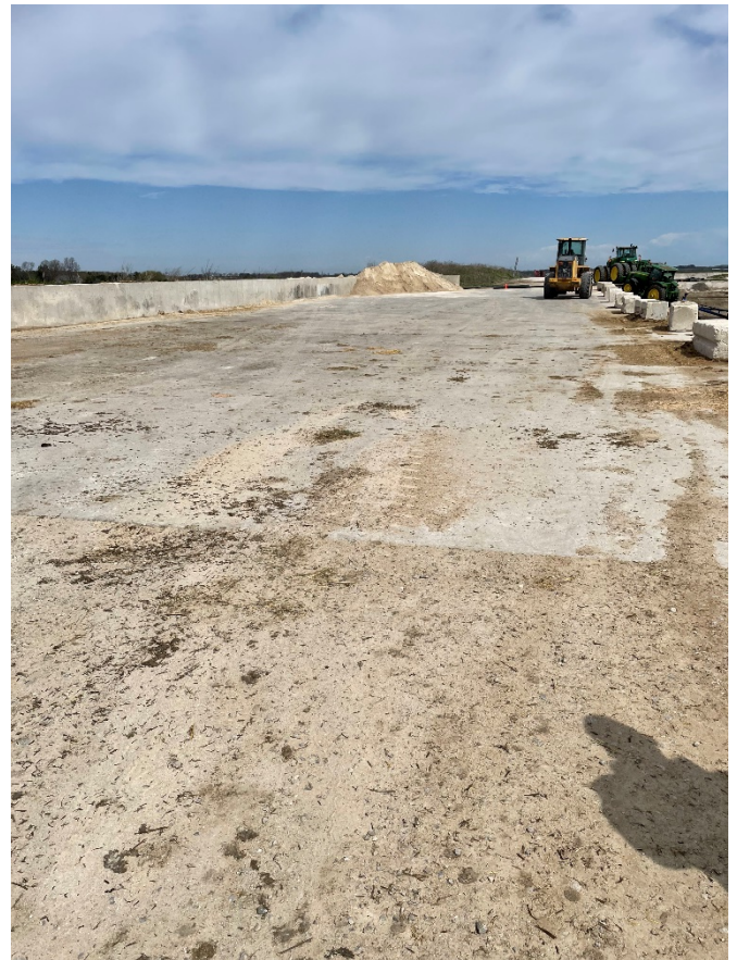
Photo 2- Solid manure stacking area west of WSF1. Photo taken facing north.
