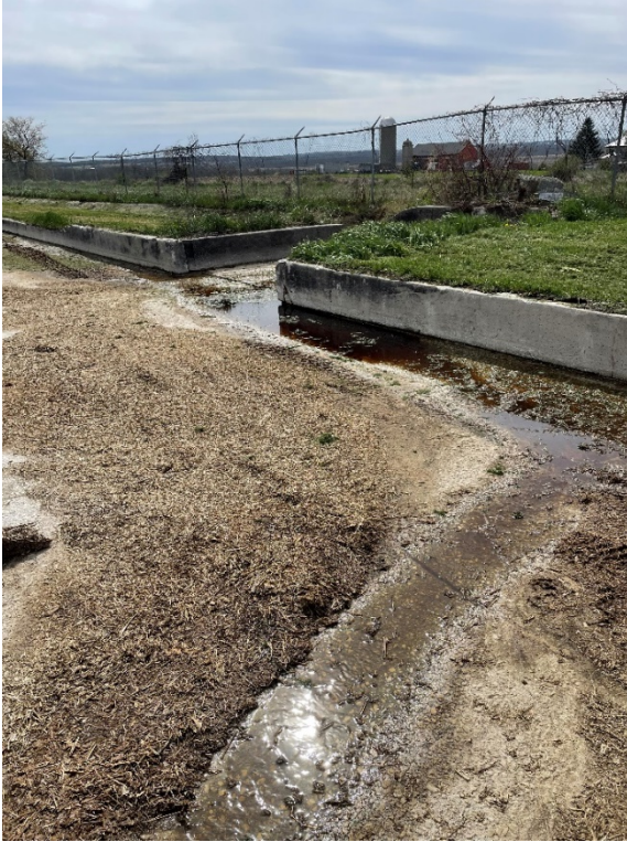
Photo 9- Feed storage area runoff control conveyance and inlet. Photo taken facing south.
