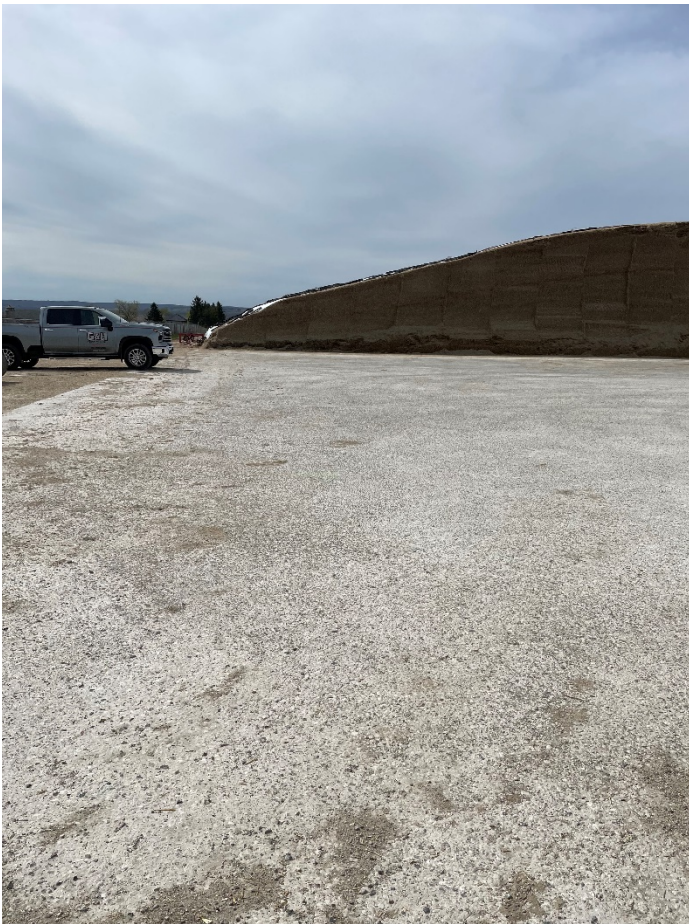
Photo 5 - Northern portion of the feed pad. Photo taken facing south.
