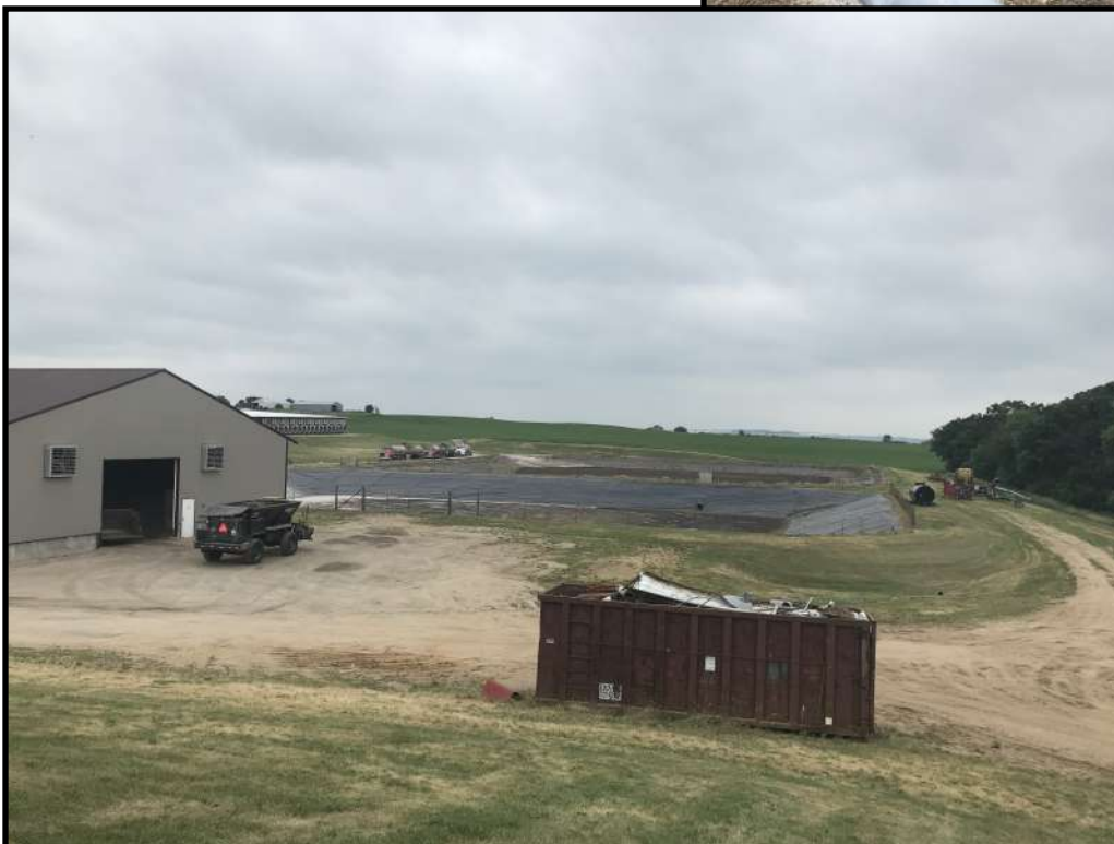
Photo 5 (bottom left): Looking west across WSF 1 and WSF 2. The connection pipe between the storages can be seen pictured in WSF 1 and the sand separation building can also be seen pictured left.
