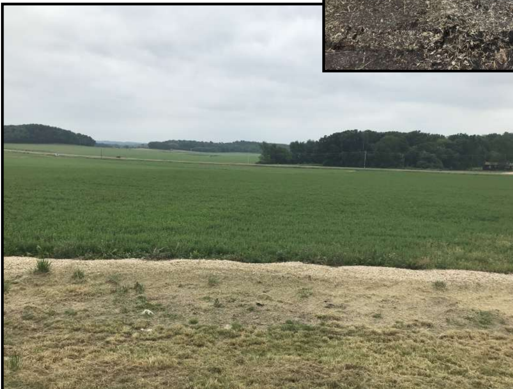
Photo 12 (bottom left): Looking south across the VTA. A gravel spreader bar has been placed at the start of the VTA and sufficient vegetative cover can be seen throughout. Only minimal vegetative burn out was observed near the beginning of the VTA.
