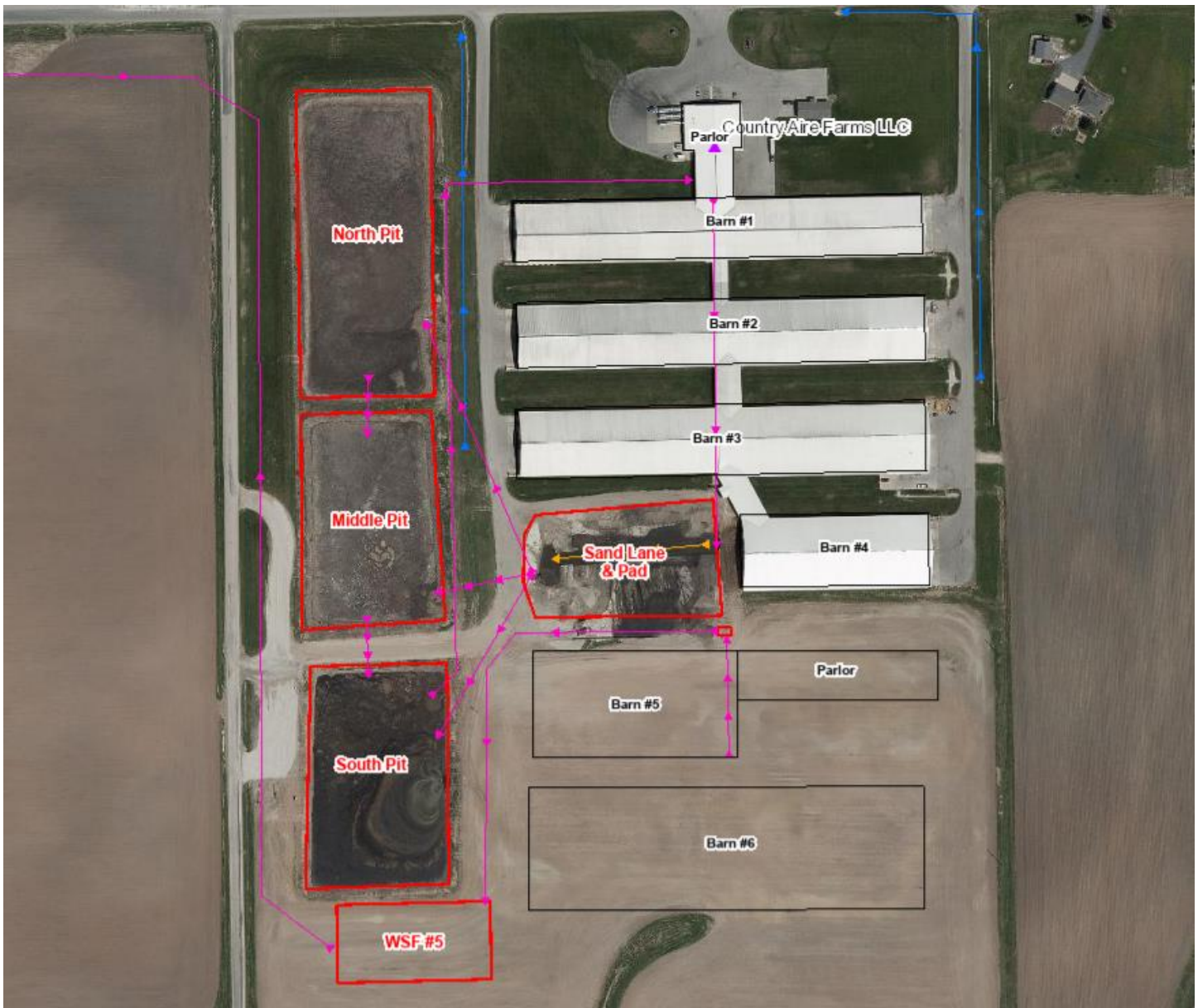
Figure 1. Aerial overview of Country Aire Farms on the south side of Lamers Clancy Road. Blue arrows indicate approximate stormwater flow paths. Yellow arrows indicate approximate contaminated runoff flow paths. Pink arrows indicate manure transfer systems.
