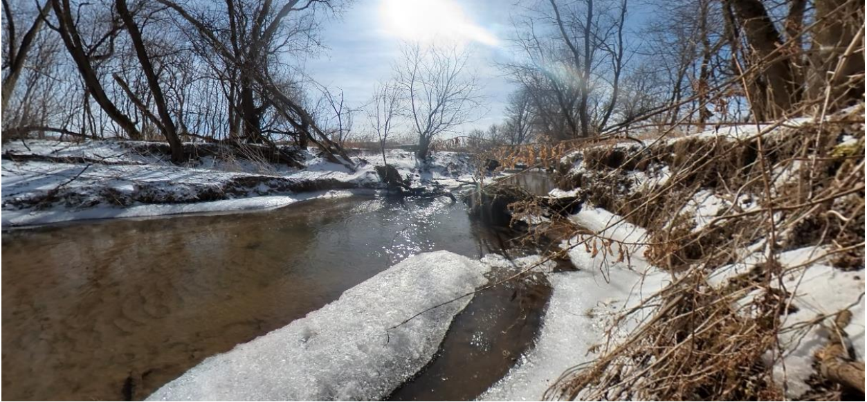
Image 9 - Severe undercut with slump, vegetative overhang, and fallen trees
