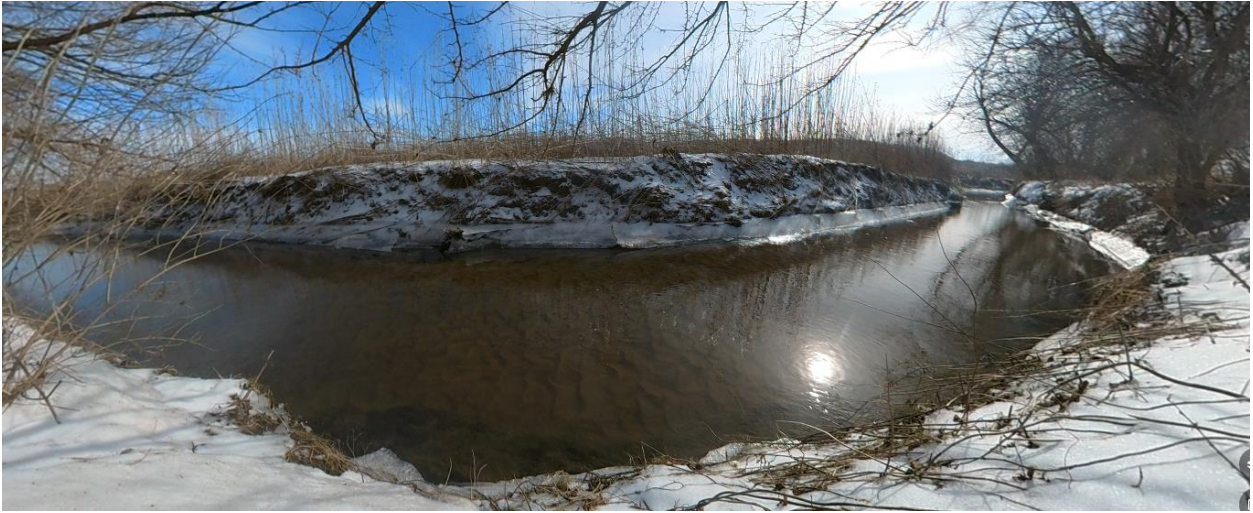
Image 3 - Severe undercut with vegetative overhang
