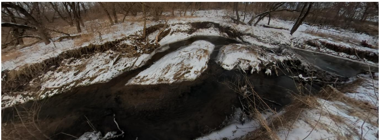
Image 14 - Severe undercut with slump, vegetative overhang, and fallen trees
