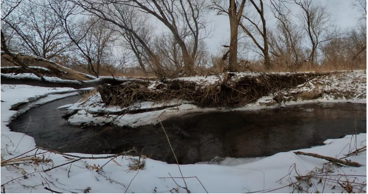
Image 15 - Severe undercut with slump, vegetative overhang, exposed roots and fallen trees
