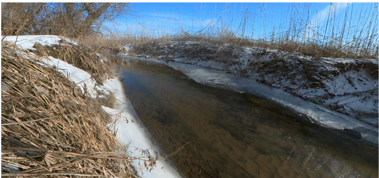
Image 2 - Severe undercut with vegetative overhang
