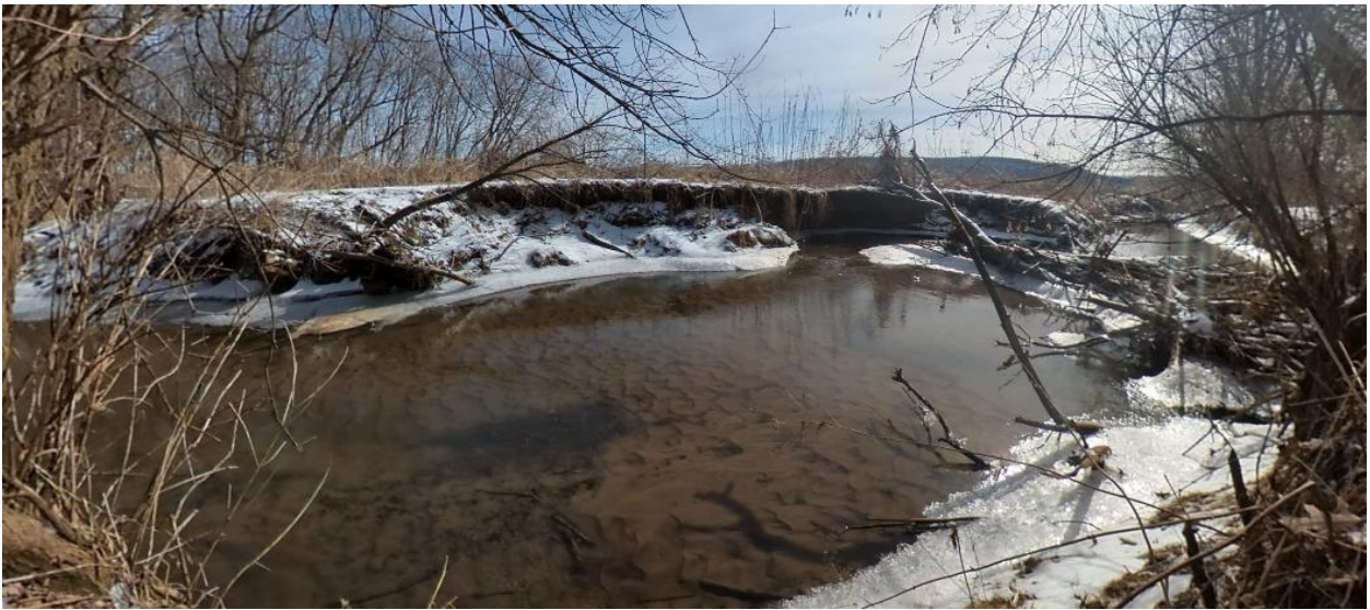
Image 8 - Severe undercut with slump, vegetative overhang, and fallen tree
