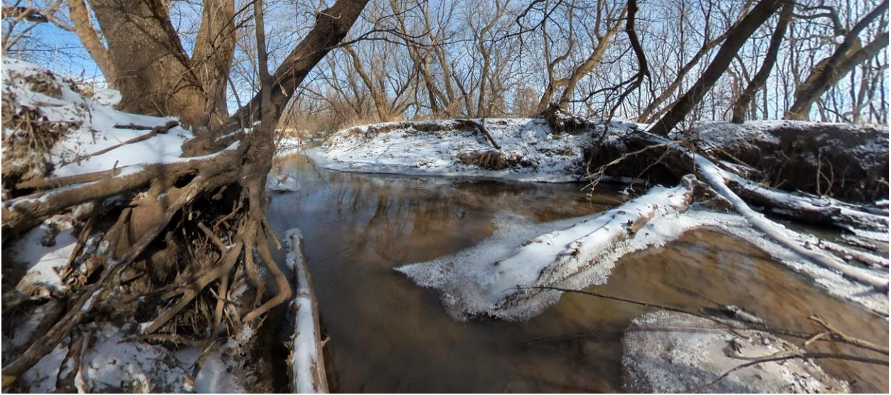
Image 11 - Severe undercut with slump, vegetative overhang, exposed roots, and fallen trees
