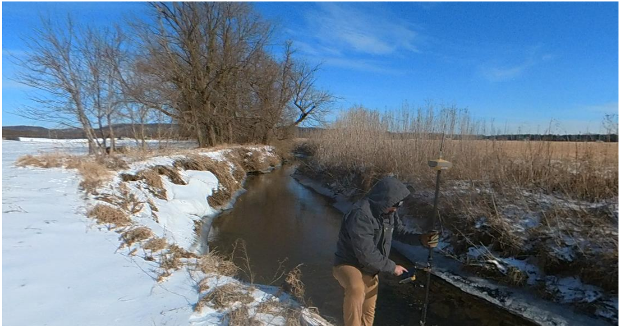
Image 1 - Severe undercut with vegetative overhang
