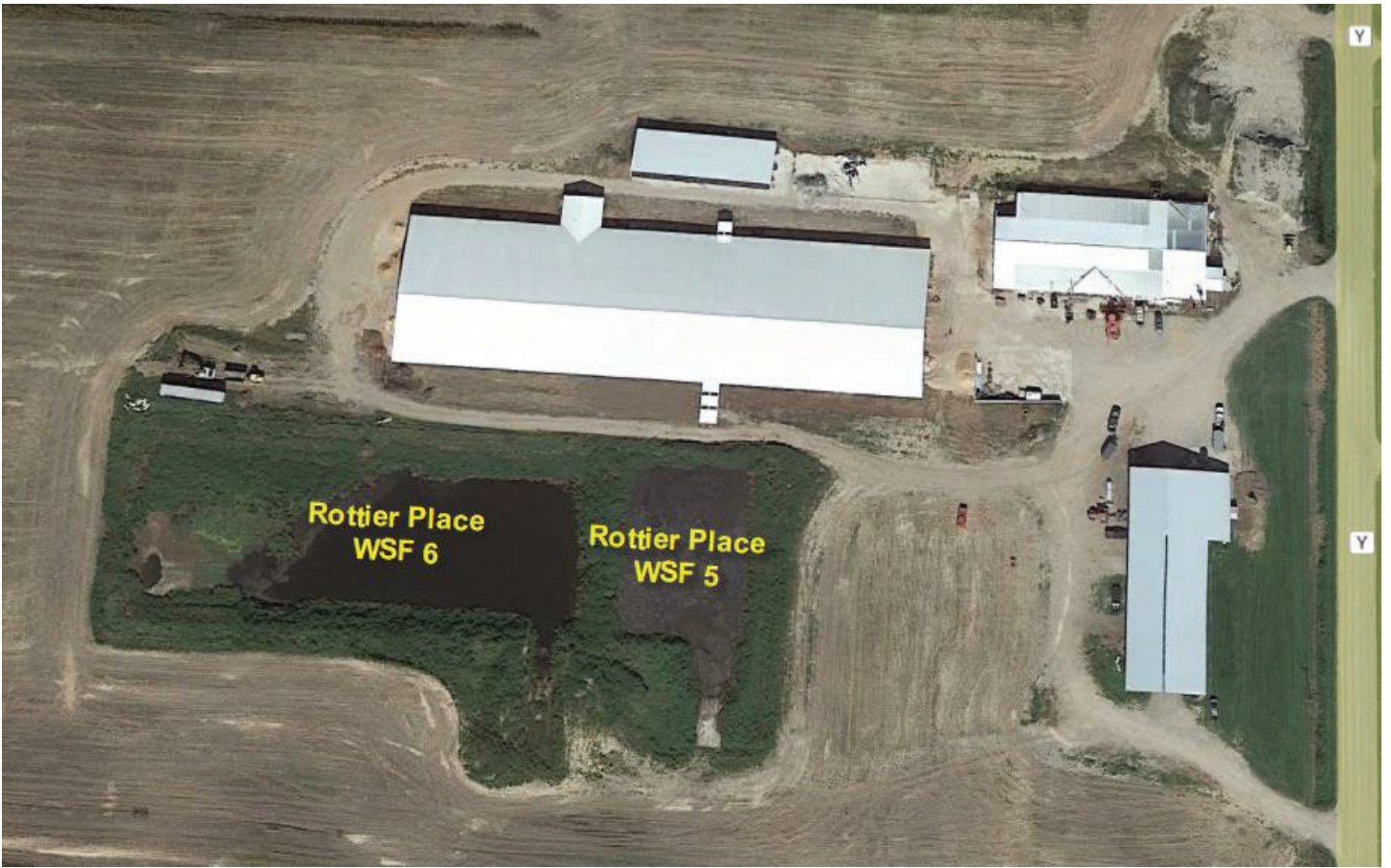
Figure 4. Aerial overview of Vandehei Farms: Rottier Place site
