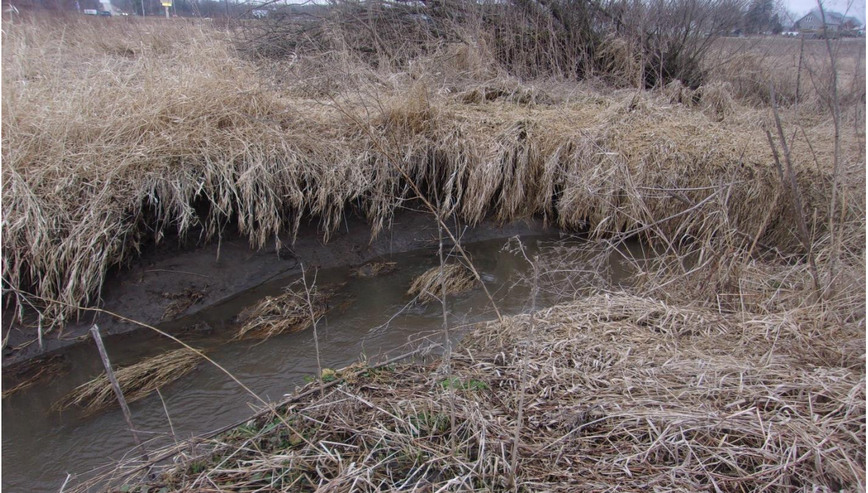
Image 5 – Severe undercut with slump and vegetative overhang.
