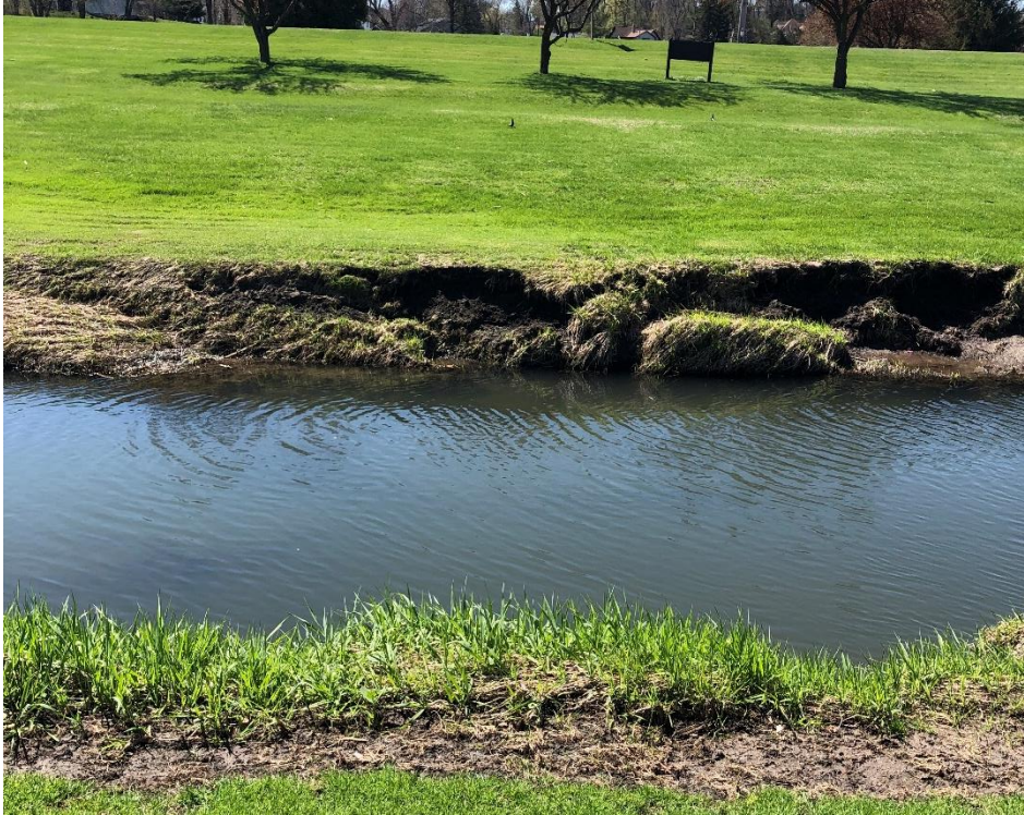
Image 19 – Severe undercut with slump and vegetative overhang.
