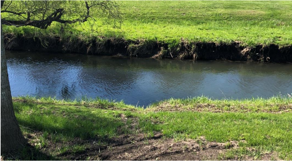
Image 18 – Severe undercut with slump and vegetative overhang.
