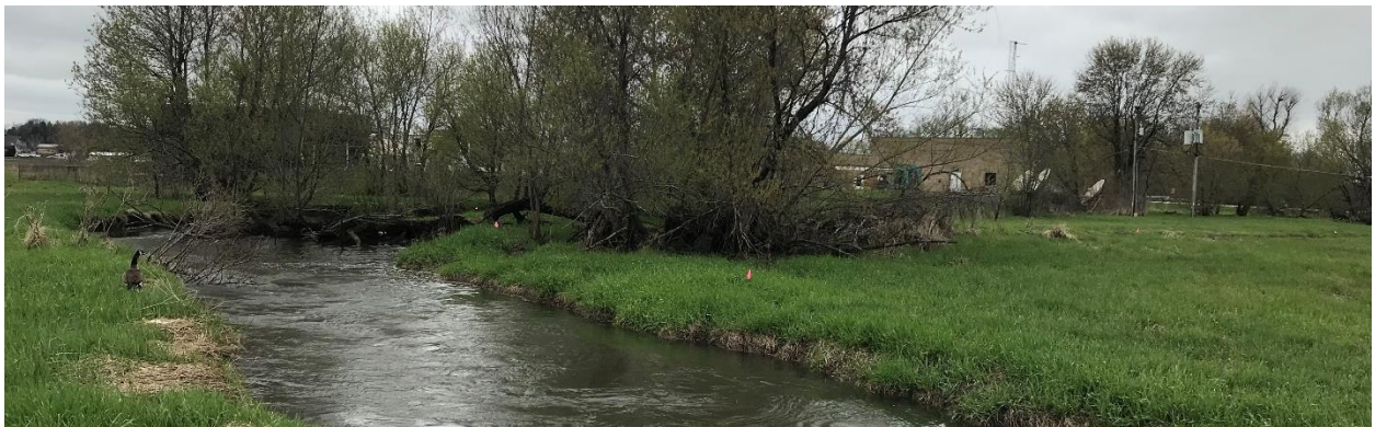
Image 24 – Severe undercut with fallen trees, exposed tree roots, and vegetative overhang.
