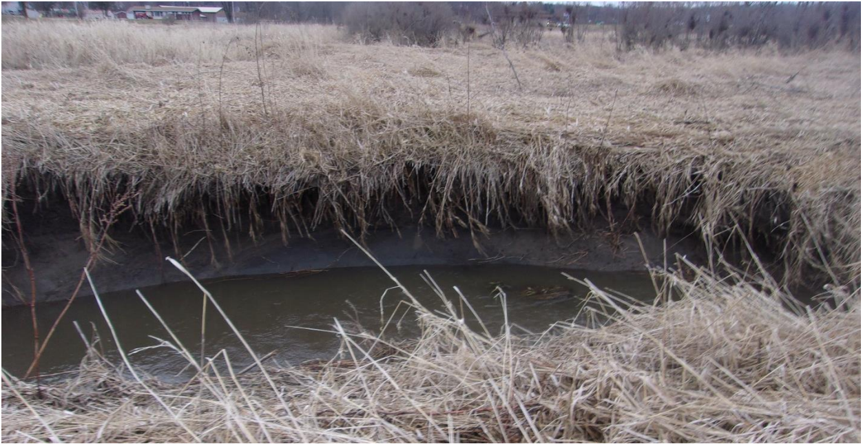
Image 6 – Severe undercut with vegetative overhang.
