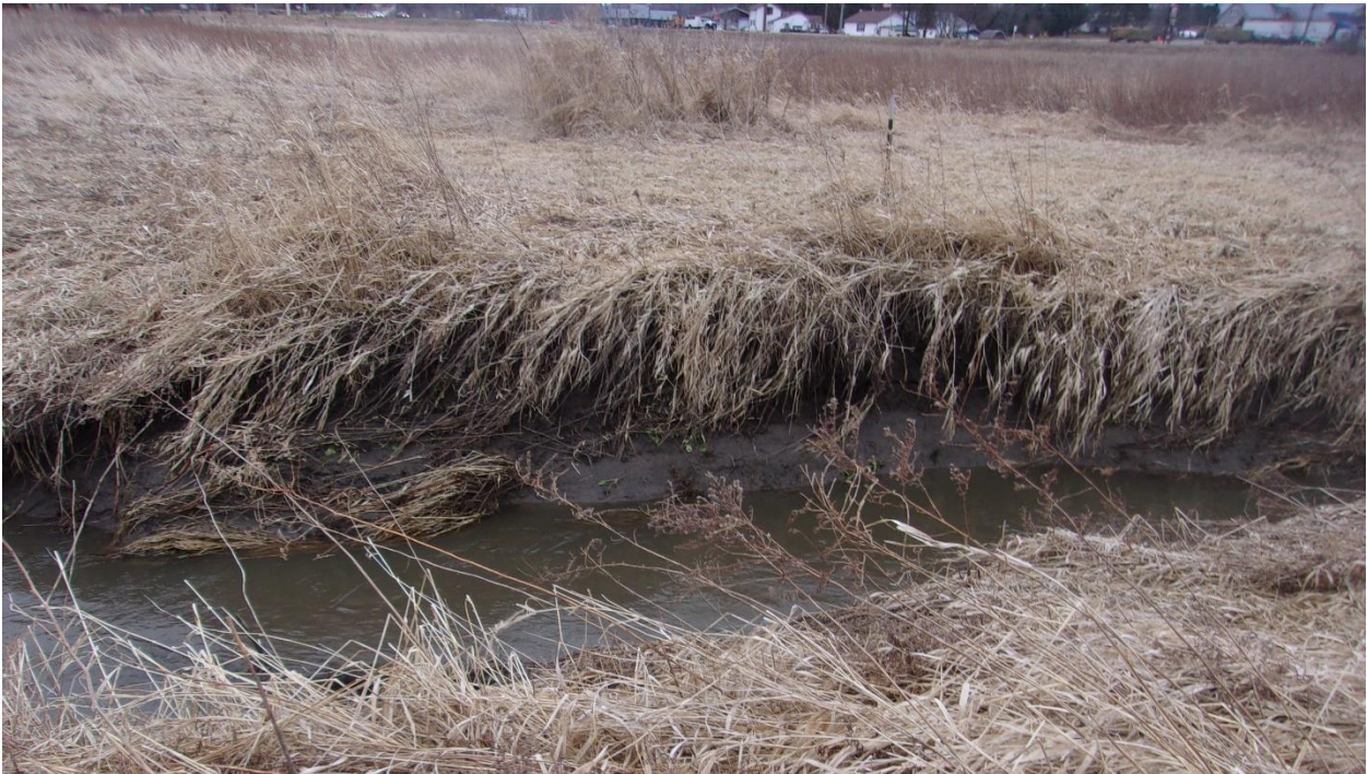
Image 2 – Severe undercut with slump and vegetative overhang.
