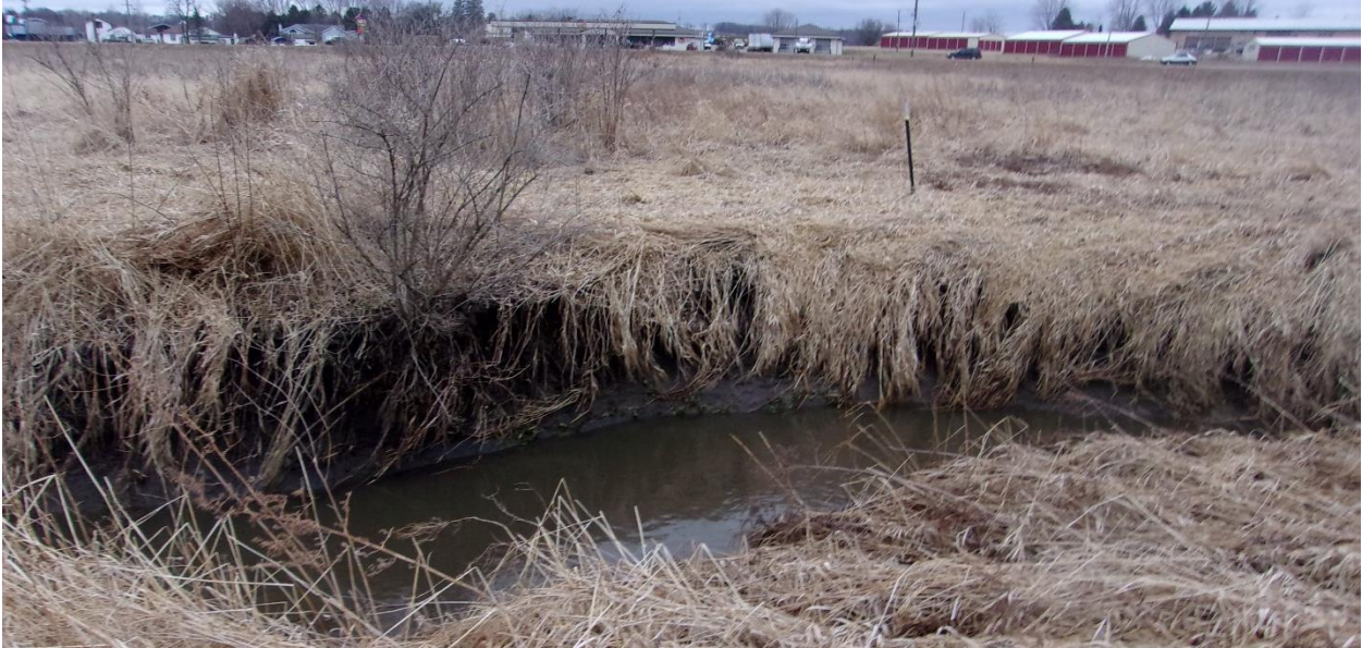
Image 1 – Sever undercut with vegetative overhang.
