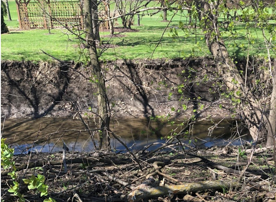
Image 13 – Severe undercut, exposed tree roots, and vegetative overhang.
