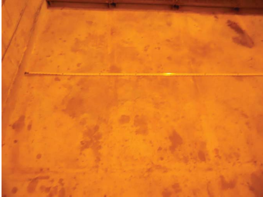
D-3 EAST - NO VISIBLE CRACKS
