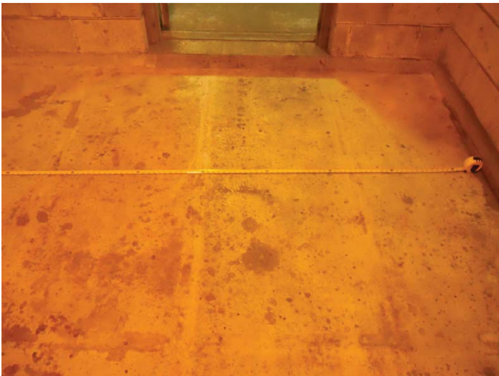
D-1 WEST - NO VISIBLE CRACKS
