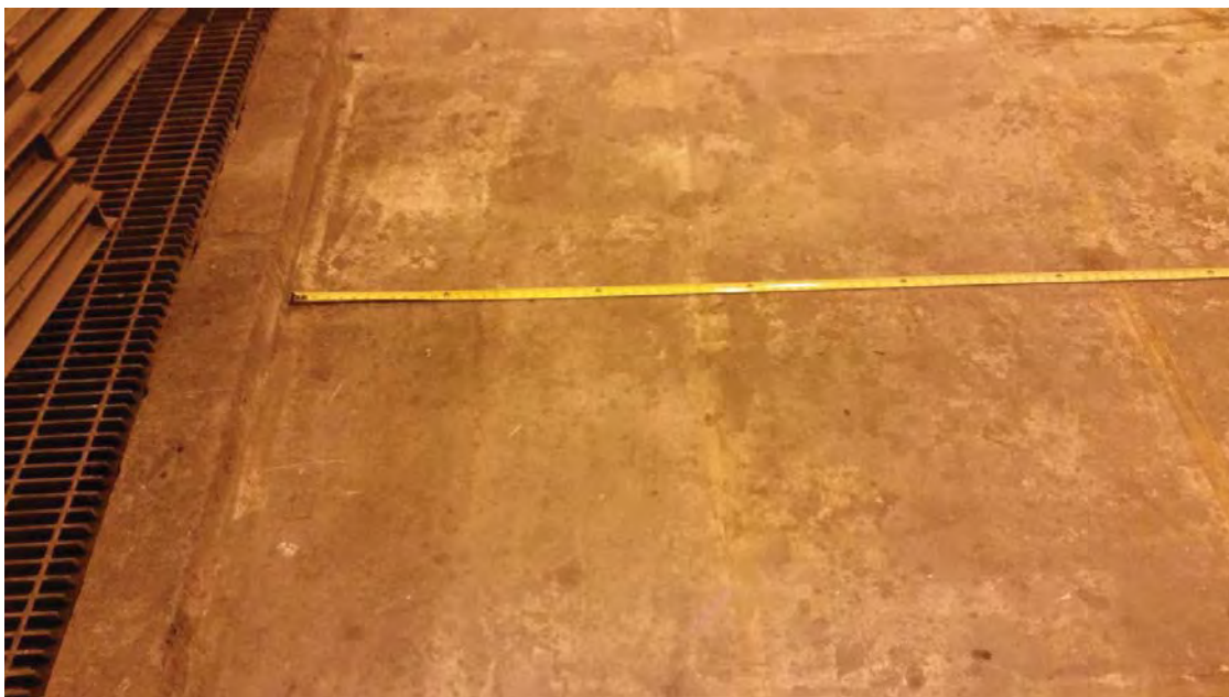
E-4 WEST (1) - NO VISIBLE CRACKS
