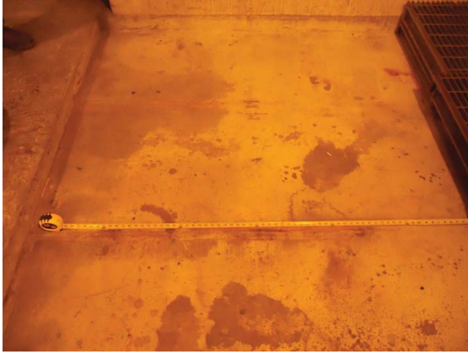
A-5 NORTH – NO VISIBLE CRACKS
