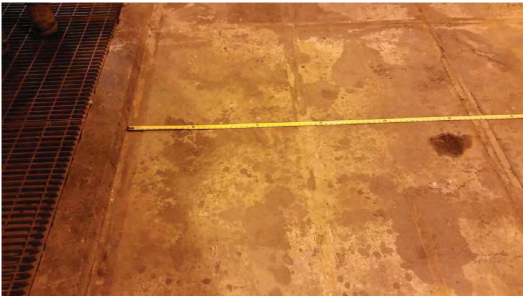
E-2 WEST (1) - NO VISIBLE CRACKS
