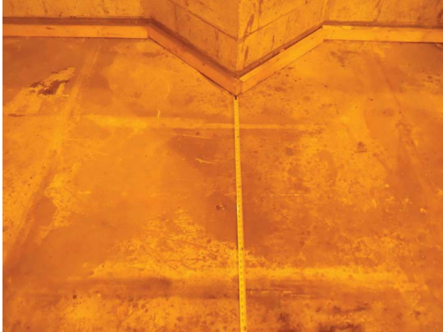
E-4 EAST (1) - NO VISIBLE CRACKS
