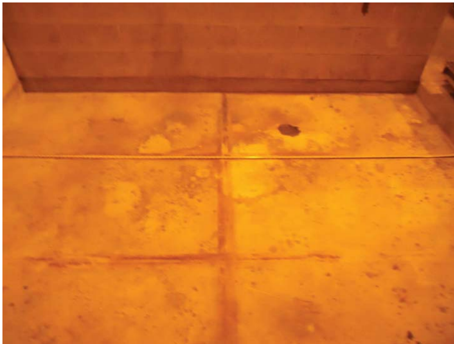
I-2 AND I-3 - NO VISIBLE CRACKS
