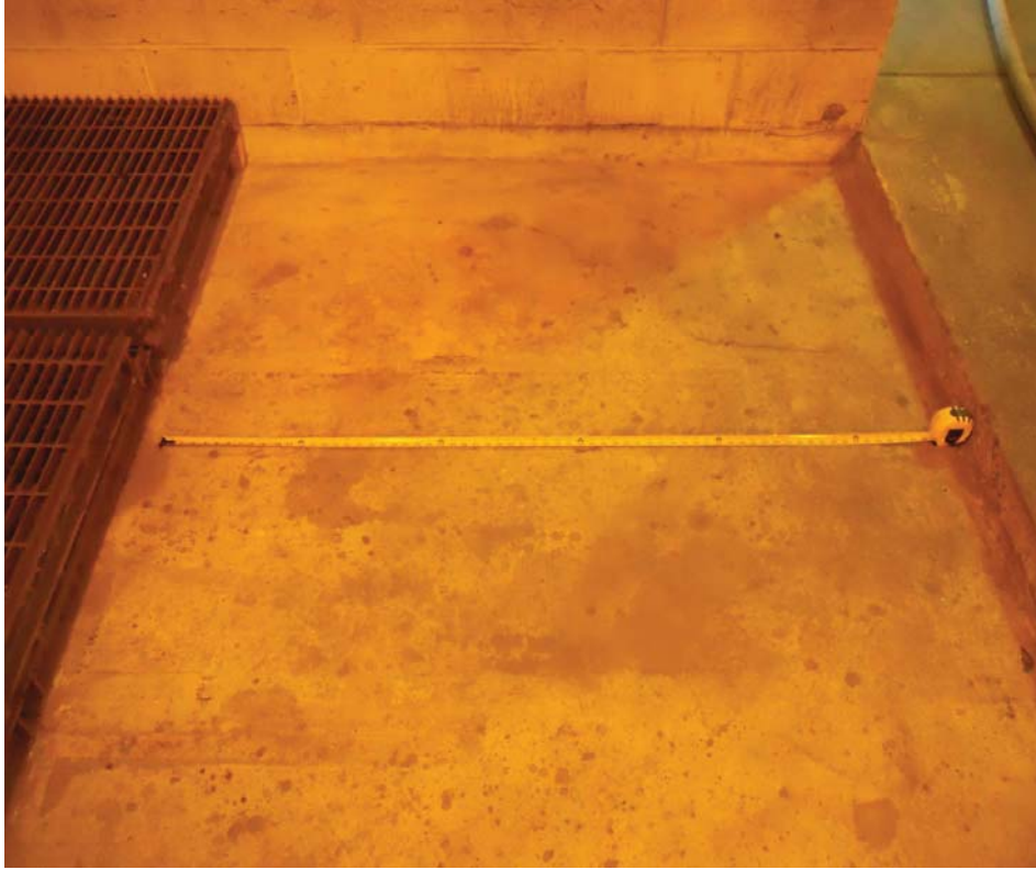
A-1 NORTH – NO VISIBLE CRACKS
