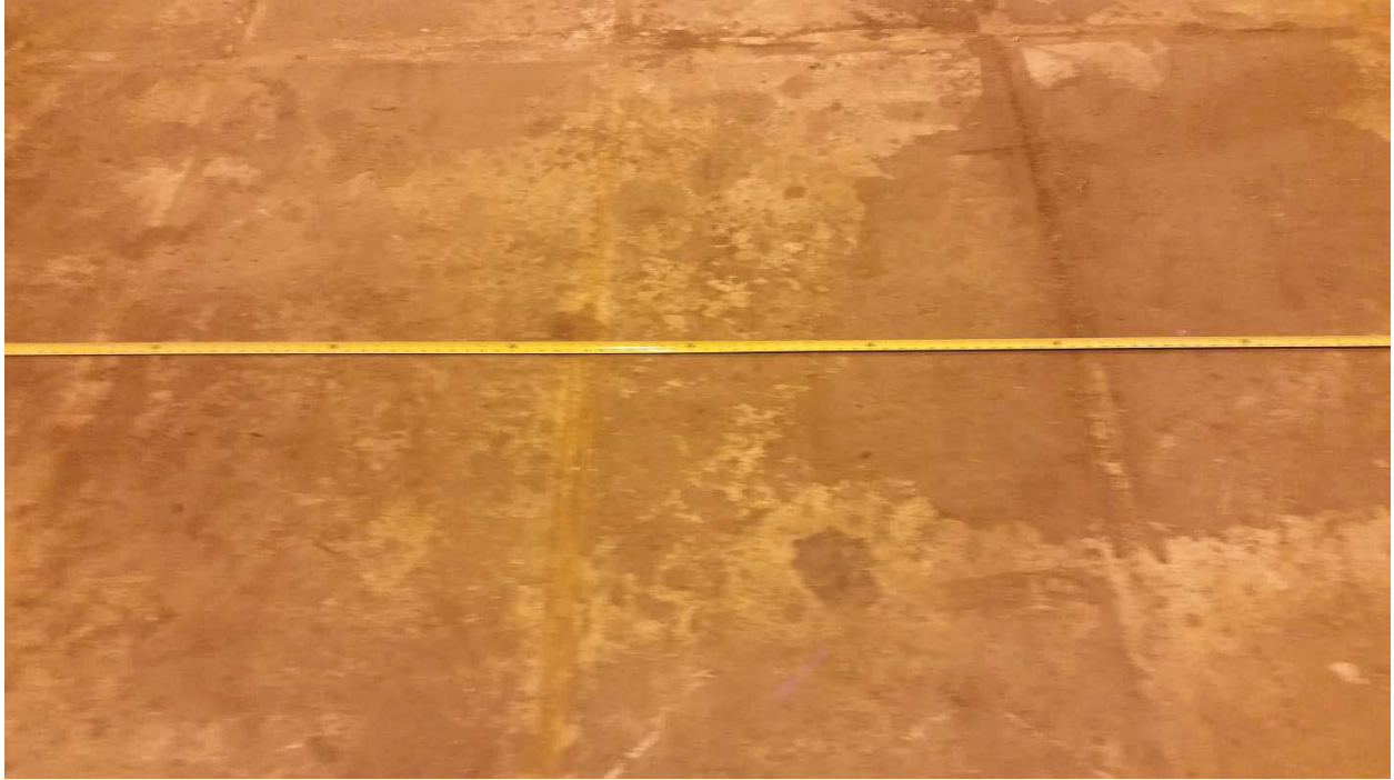
E-4 WEST (2) - NO VISIBLE CRACKS
