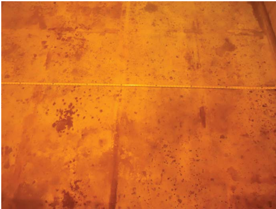
D-2 WEST - NO VISIBLE CRACKS
