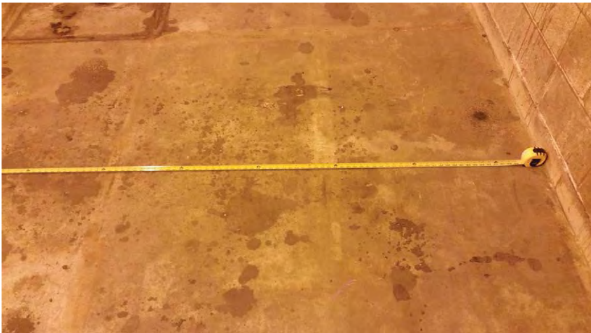
E-3 WEST (3) - NO VISIBLE CRACKS
