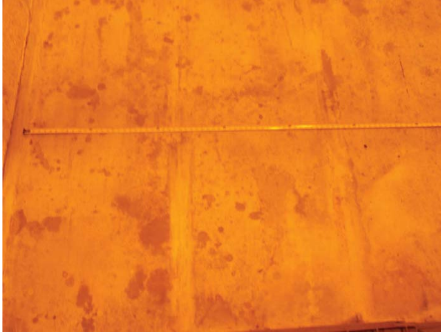
D-4 EAST - NO VISIBLE CRACKS
