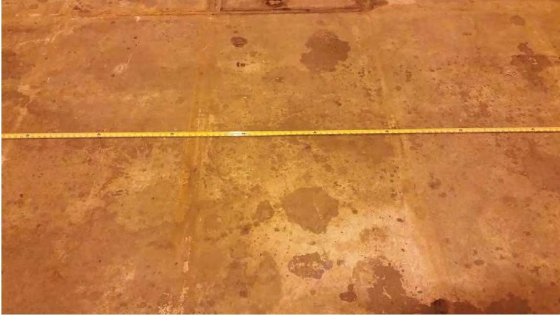
E-3 WEST (2) - NO VISIBLE CRACKS
