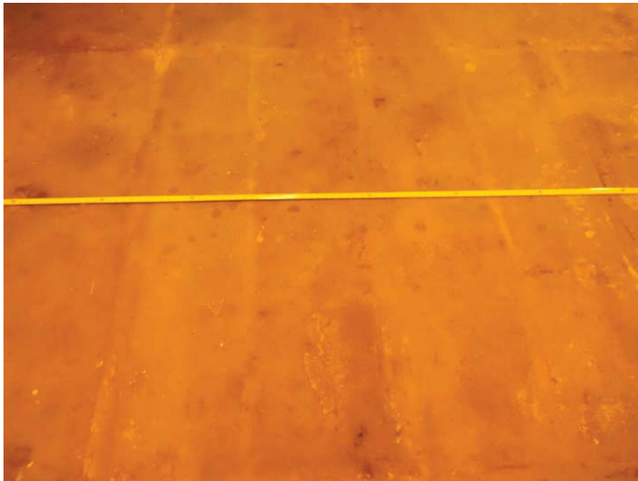
E-2 EAST (2) - NO VISIBLE CRACKS
