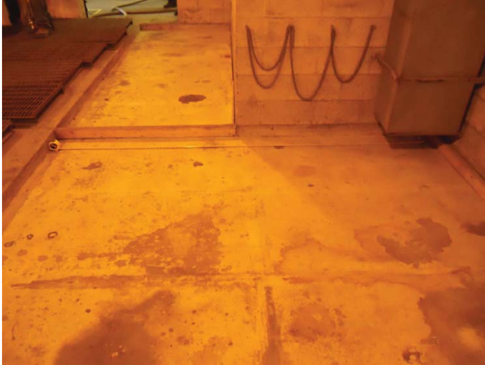
B-3 EAST - NO VISIBLE CRACKS
