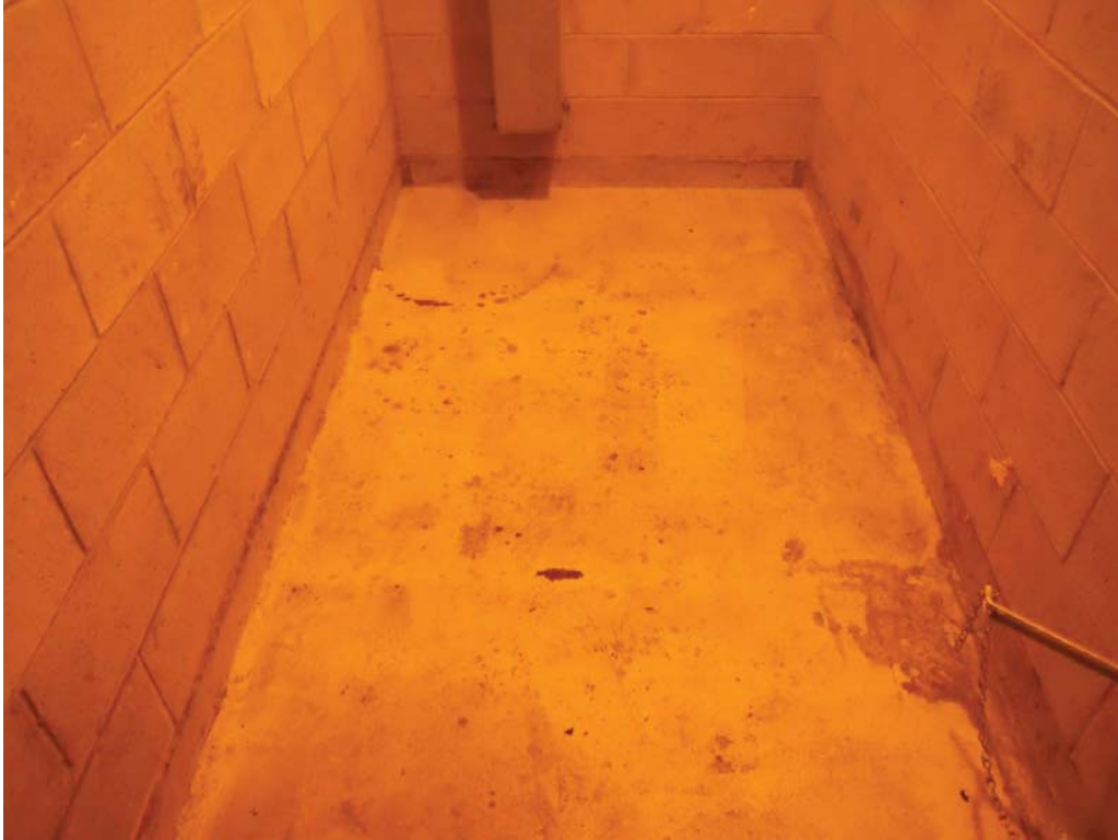
C-1 EAST - NO VISIBLE CRACKS
