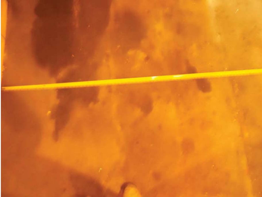
E-1 EAST (1) - NO VISIBLE CRACKS
