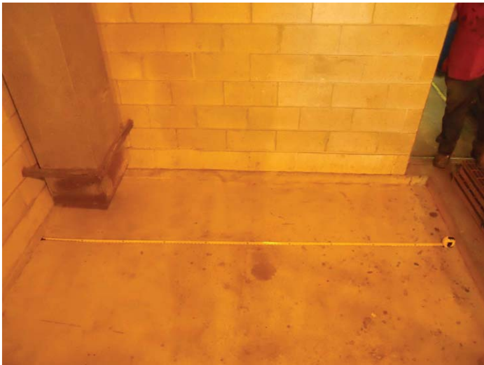
K-2 AND K-3 - NO VISIBLE CRACKS
