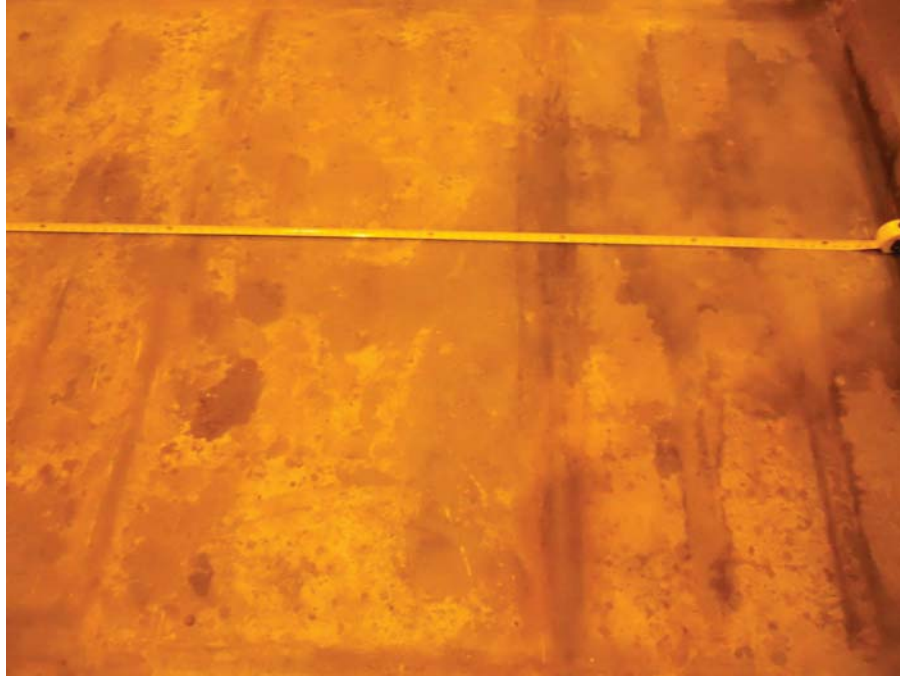
E-4 EAST (3) - NO VISIBLE CRACKS
