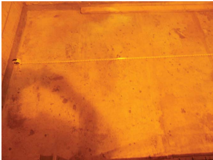
D-5 WEST - NO VISIBLE CRACKS
