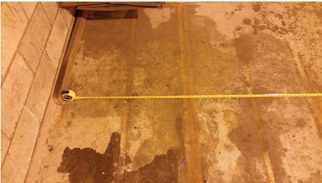
E-5 WEST (3) - NO VISIBLE CRACKS
