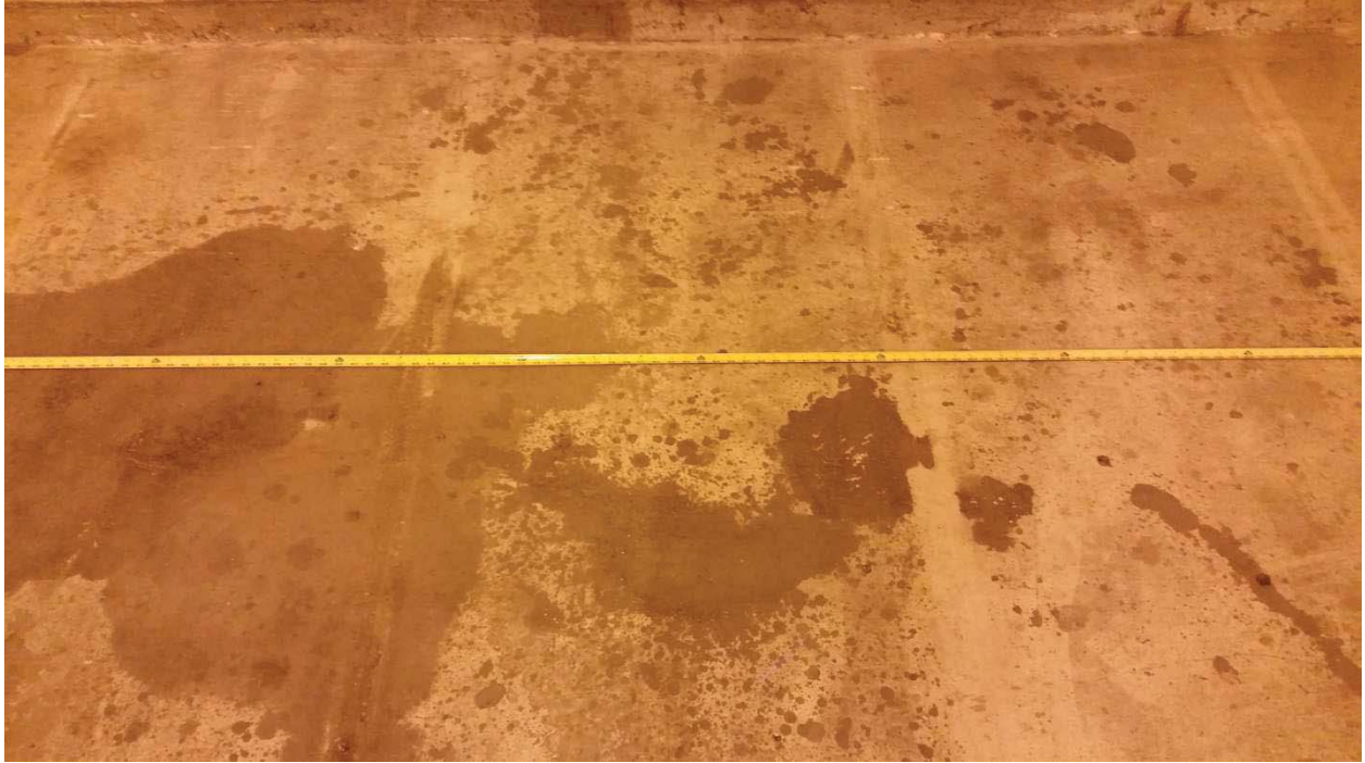
E-1 WEST (2) - NO VISIBLE CRACKS
