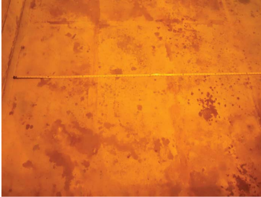
D-2 EAST - NO VISIBLE CRACKS
