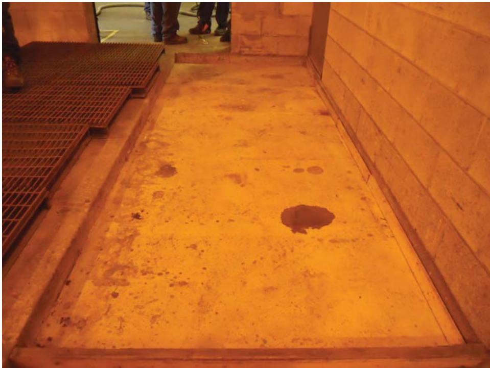
B-3 WEST - NO VISIBLE CRACKS
