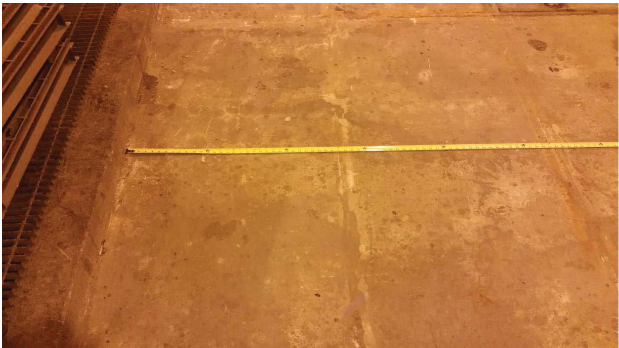
E-3 WEST (1) - NO VISIBLE CRACKS
