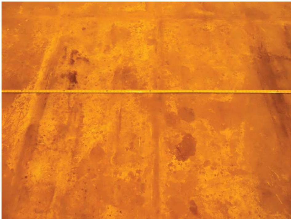
E-4 EAST (2) - NO VISIBLE CRACKS
