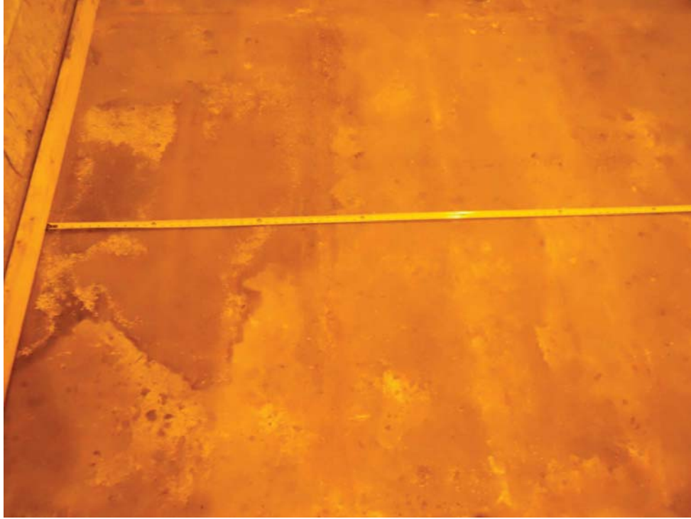
E-3 EAST (1) - NO VISIBLE CRACKS
