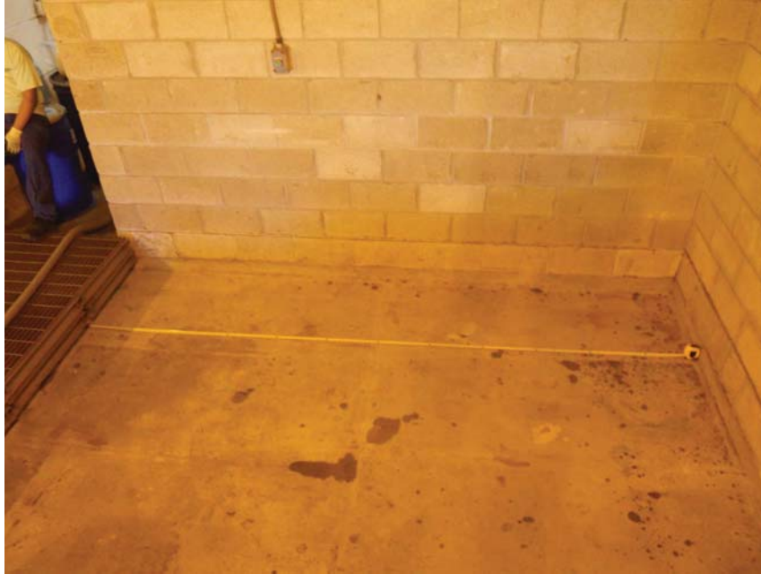
F-1 AND F-2 - NO VISIBLE CRACKS
