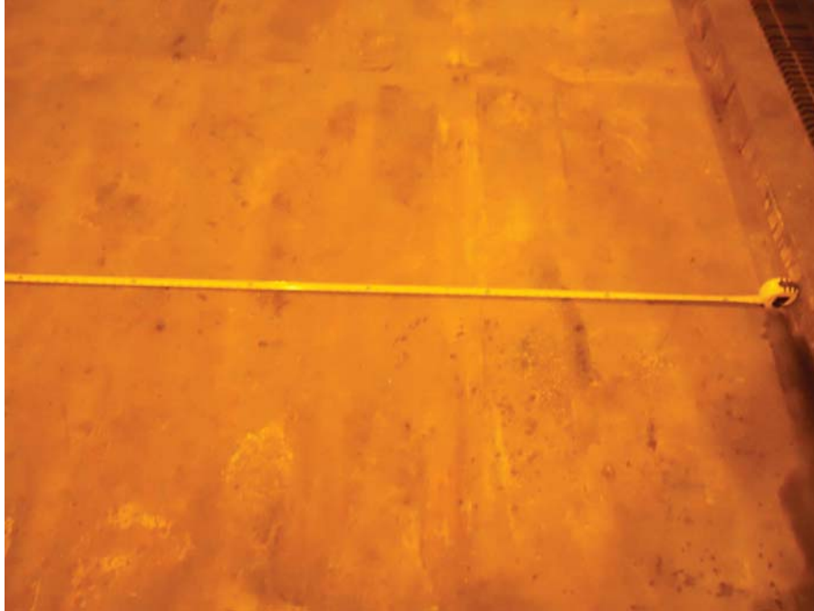
E-3 EAST (3) - NO VISIBLE CRACKS
