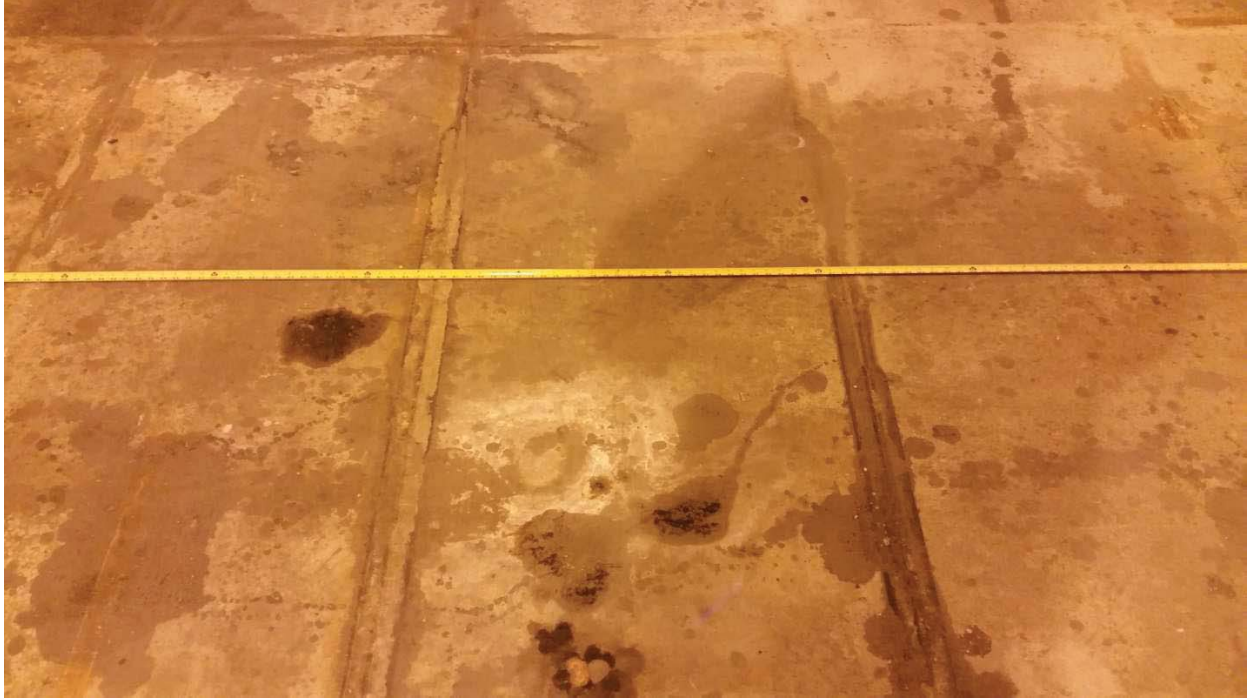
E-2 WEST (2) - NO VISIBLE CRACKS
