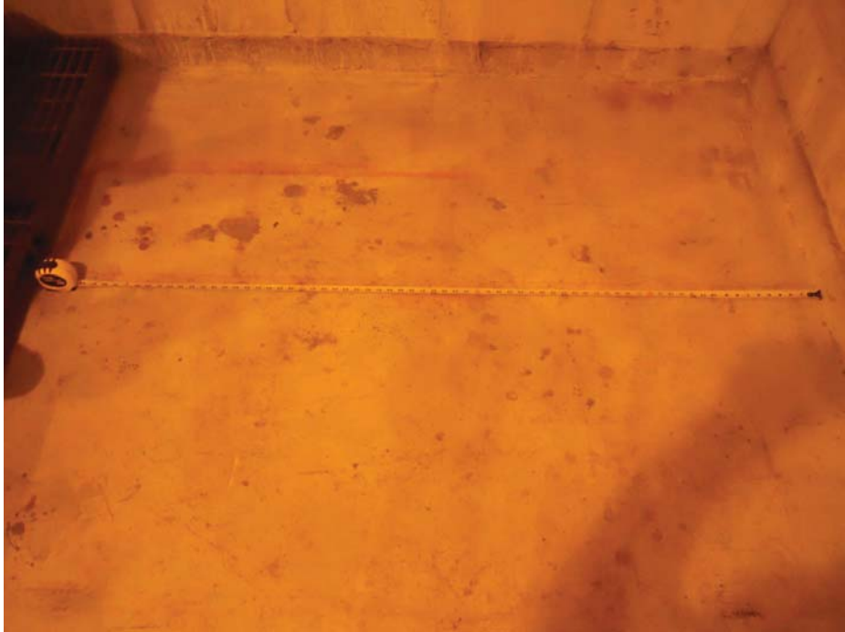
A-5 SOUTH - NO VISIBLE CRACKS
