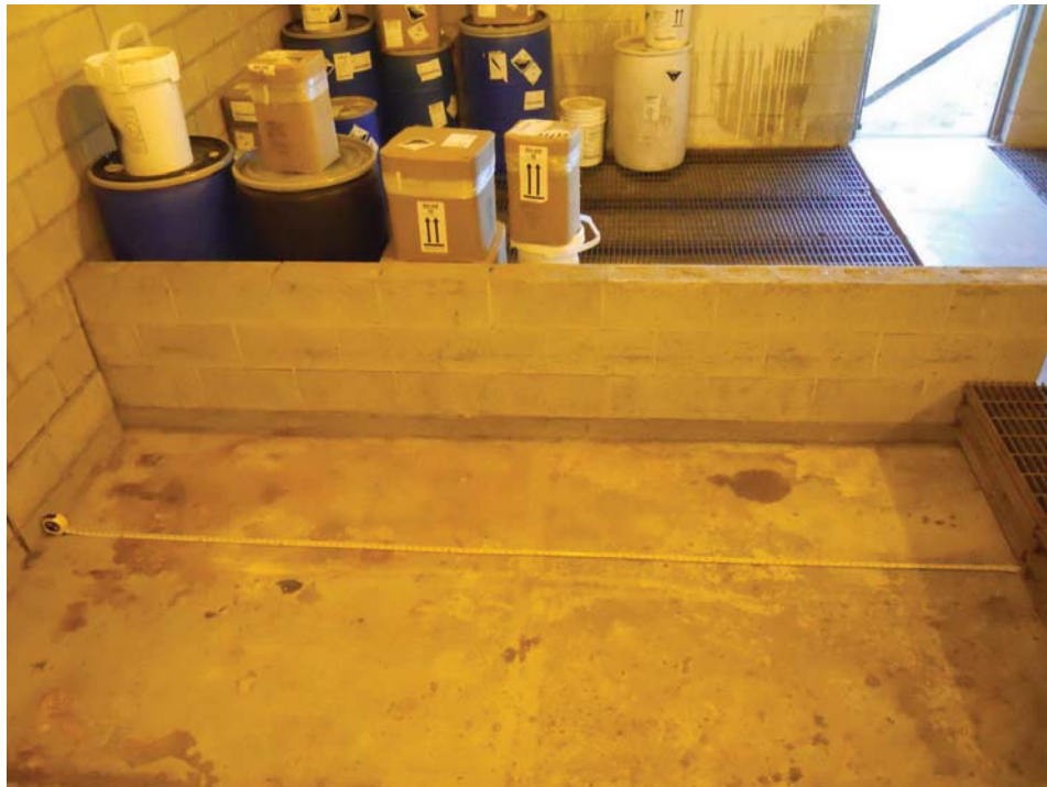
G-2 AND G-3 - NO VISIBLE CRACKS
