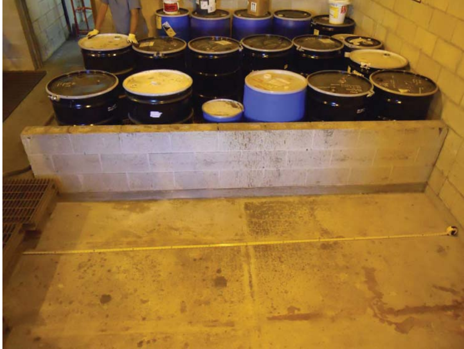
G-1 AND G-2 - NO VISIBLE CRACKS
