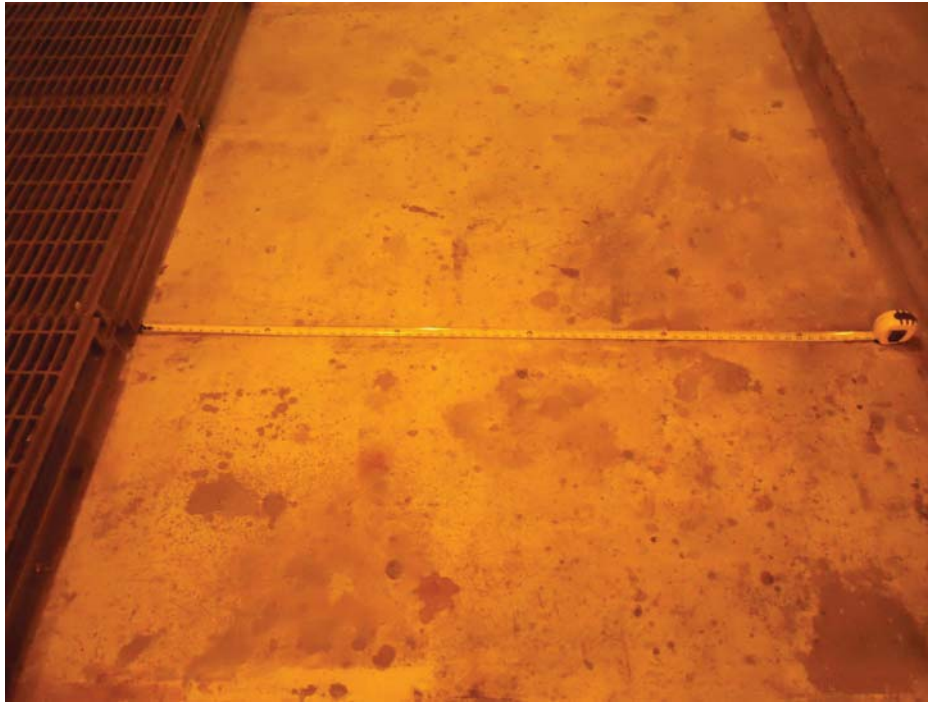
A-2 NORTH - NO VISIBLE CRACKS
