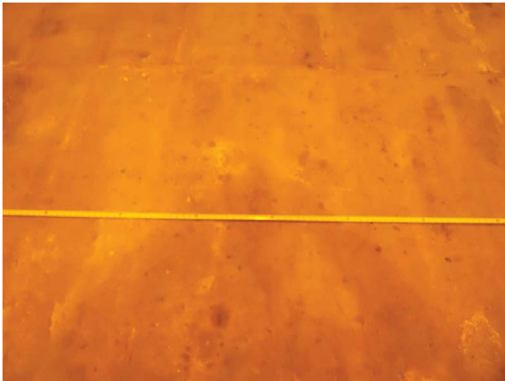
E-3 EAST (2) - NO VISIBLE CRACKS
