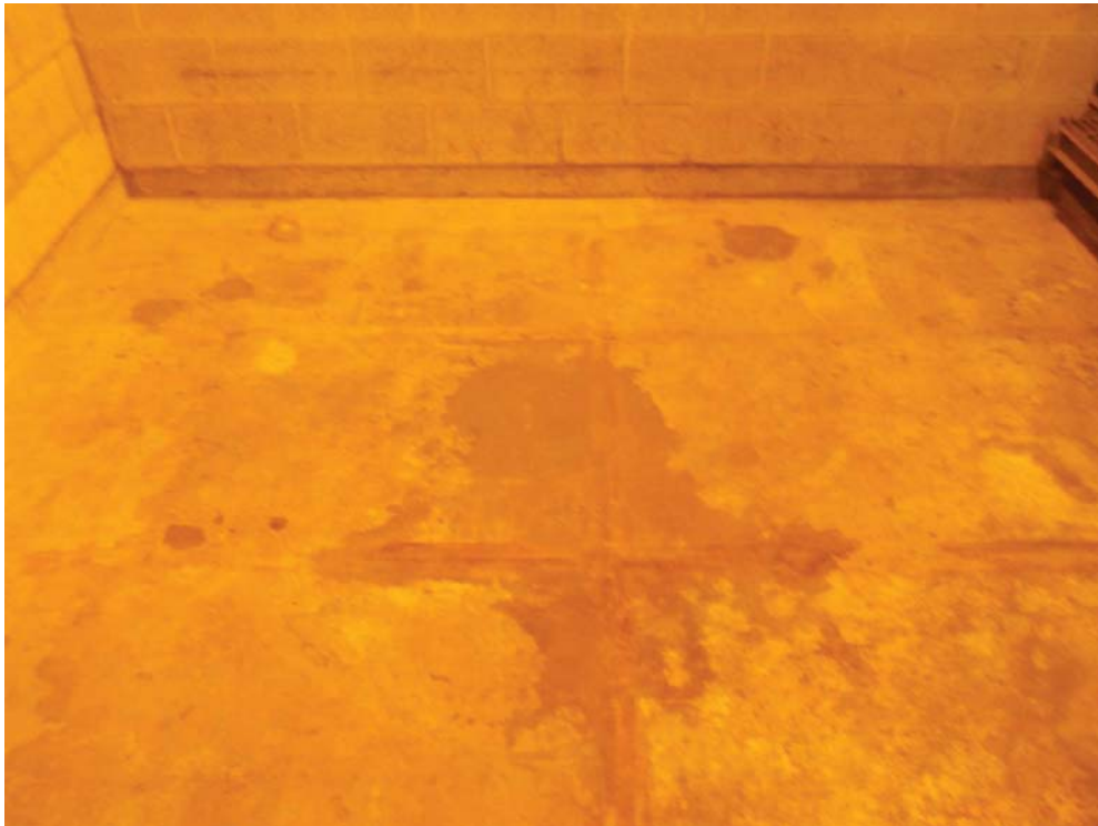
J-2 AND J-3 - NO VISIBLE CRACKS
