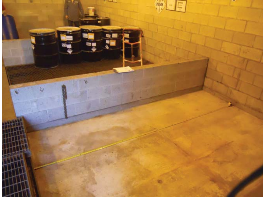
H-1 AND H-2 - NO VISIBLE CRACKS
