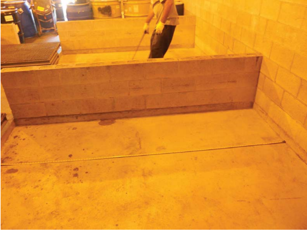
K-1 AND K-2 - NO VISIBLE CRACKS
