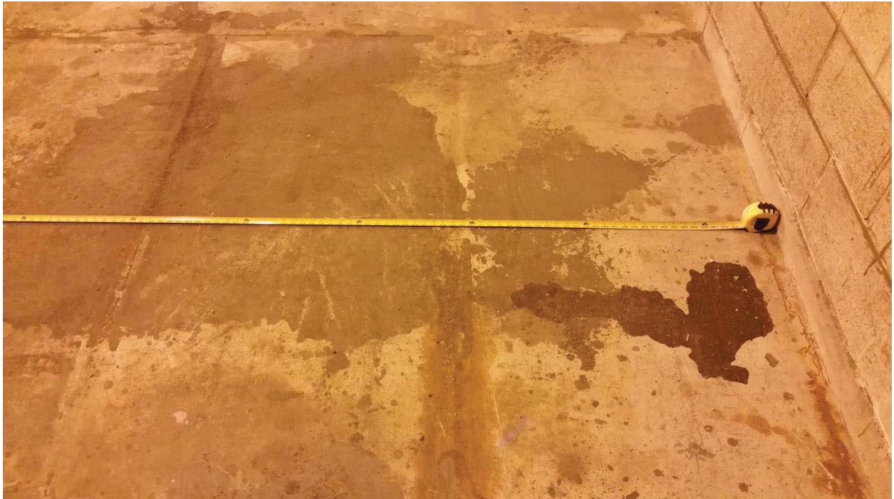
E-4 WEST (3) - NO VISIBLE CRACKS
