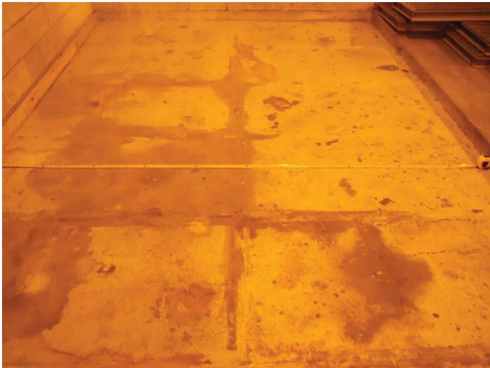
B-2 - NO VISIBLE CRACKS
