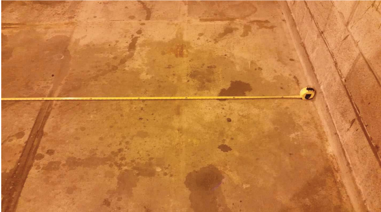
E-2 WEST (3) - NO VISIBLE CRACKS
