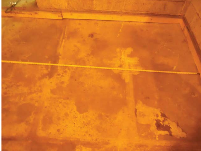
E-5 EAST (1) - NO VISIBLE CRACKS
