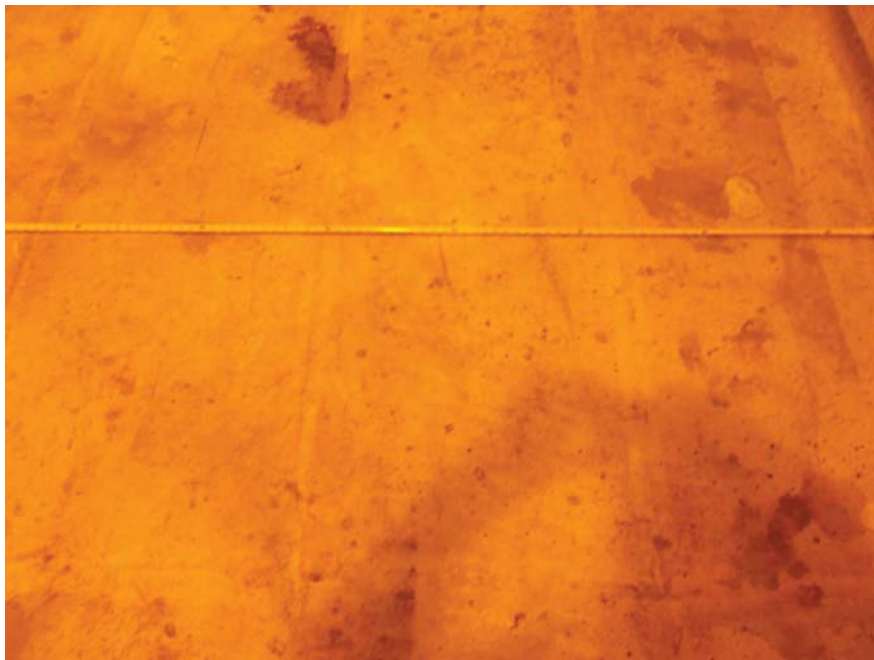
D-3 WEST - NO VISIBLE CRACKS
