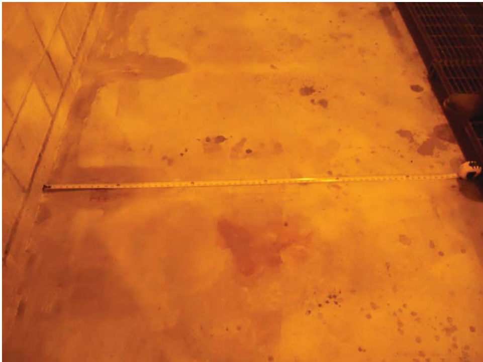
A-3 SOUTH - NO VISIBLE CRACKS
