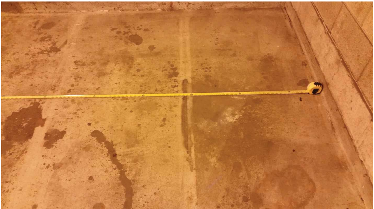
E-1 WEST (3) - NO VISIBLE CRACKS
