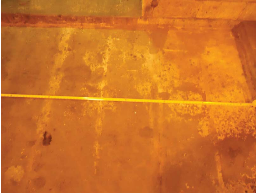
E-1 EAST (3) - NO VISIBLE CRACKS
