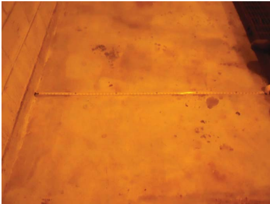
A-4 SOUTH - NO VISIBLE CRACKS
