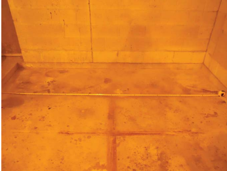
I-1 AND I-2 - NO VISIBLE CRACKS
