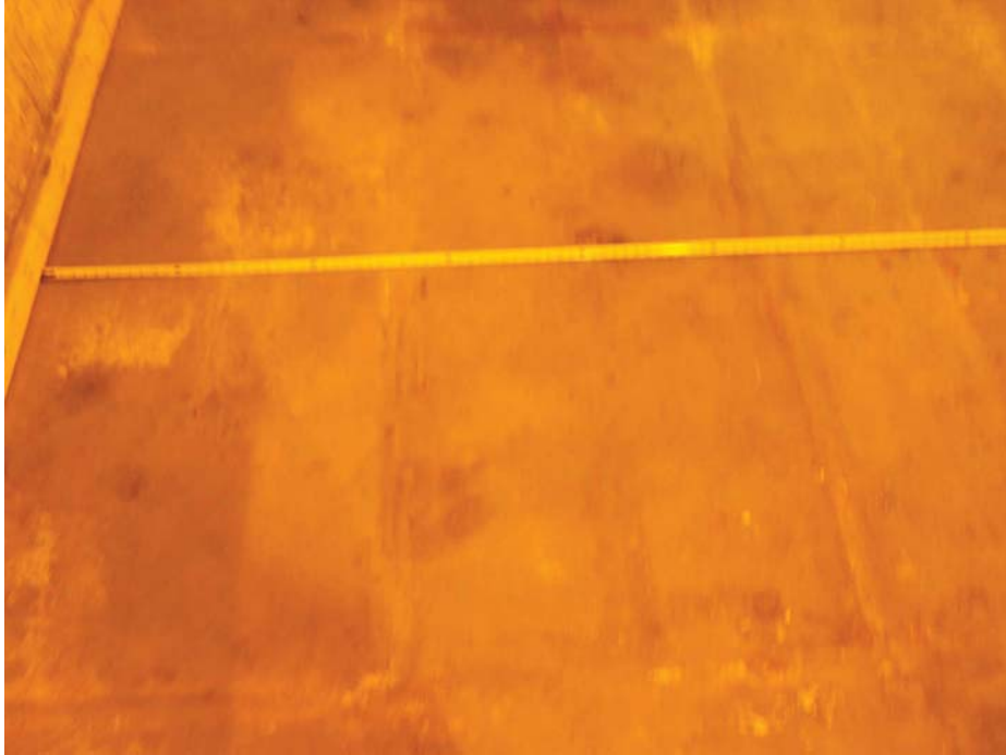
E-2 EAST (1) - NO VISIBLE CRACKS
