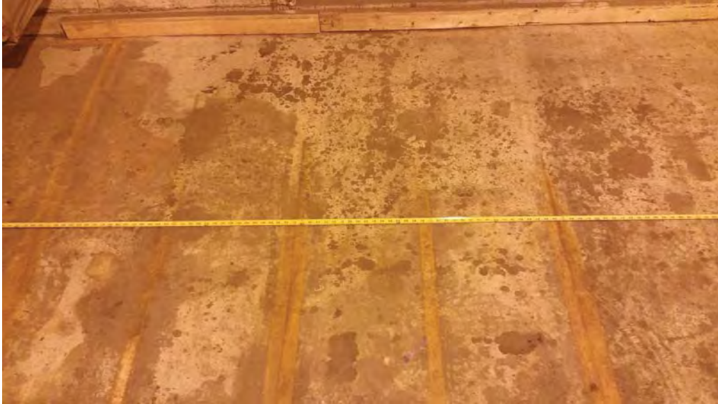
E-5 WEST (2) - NO VISIBLE CRACKS
