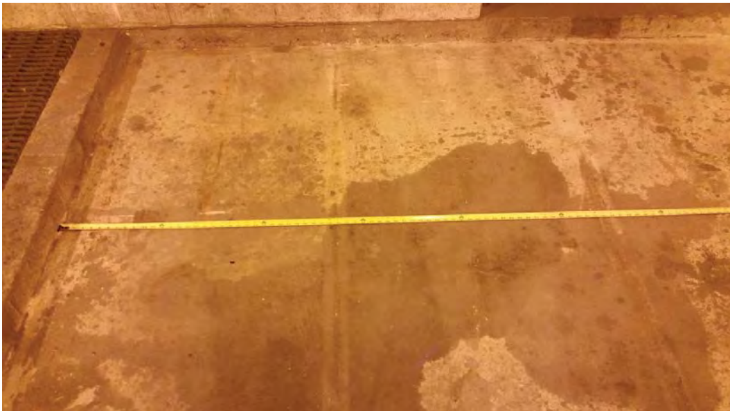
E-1 WEST (1) - NO VISIBLE CRACKS
