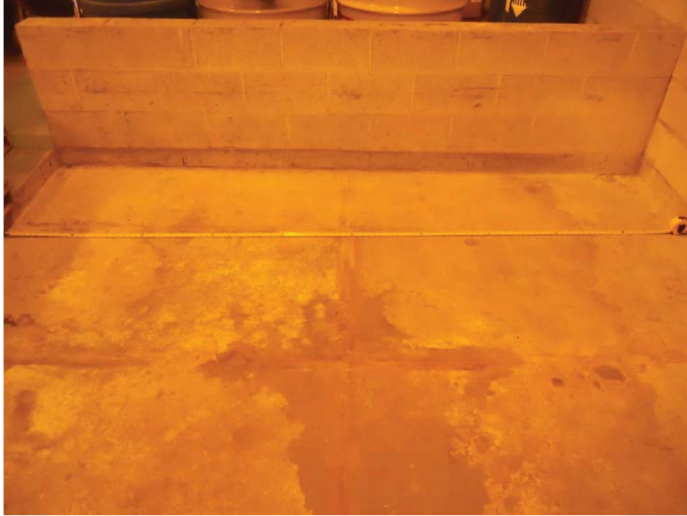
J-1 AND J-2 - NO VISIBLE CRACKS
