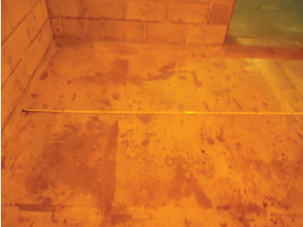
D-1 EAST - NO VISIBLE CRACKS
