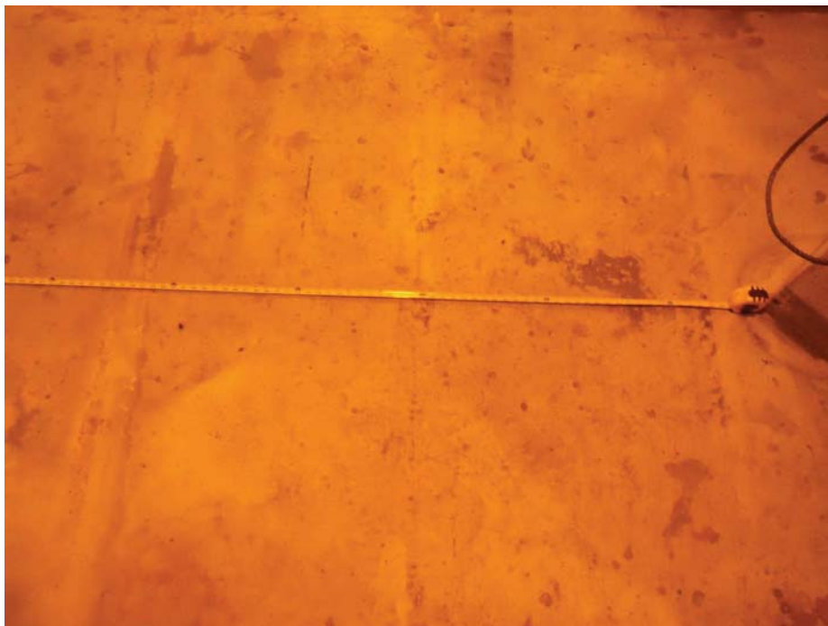
D-4 WEST - NO VISIBLE CRACKS
