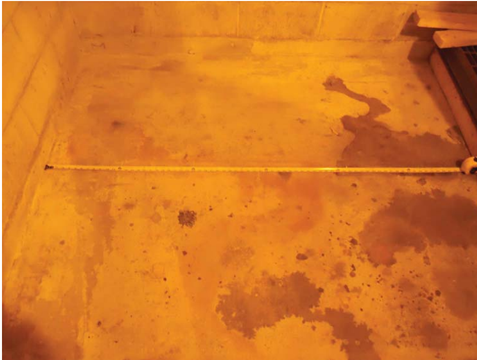
A-1 SOUTH – NO VISIBLE CRACKS
