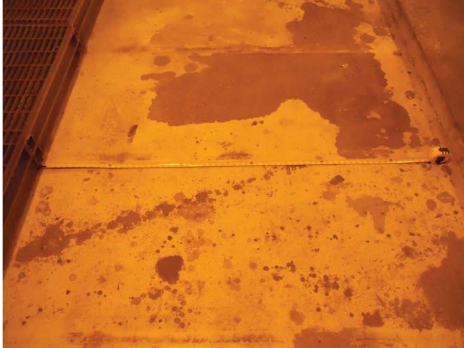
A-4 NORTH - NO VISIBLE CRACKS
