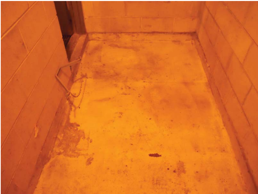
C-1 WEST - NO VISIBLE CRACKS
