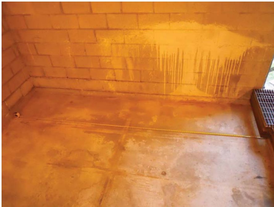
H-2 AND H-3 - NO VISIBLE CRACKS
