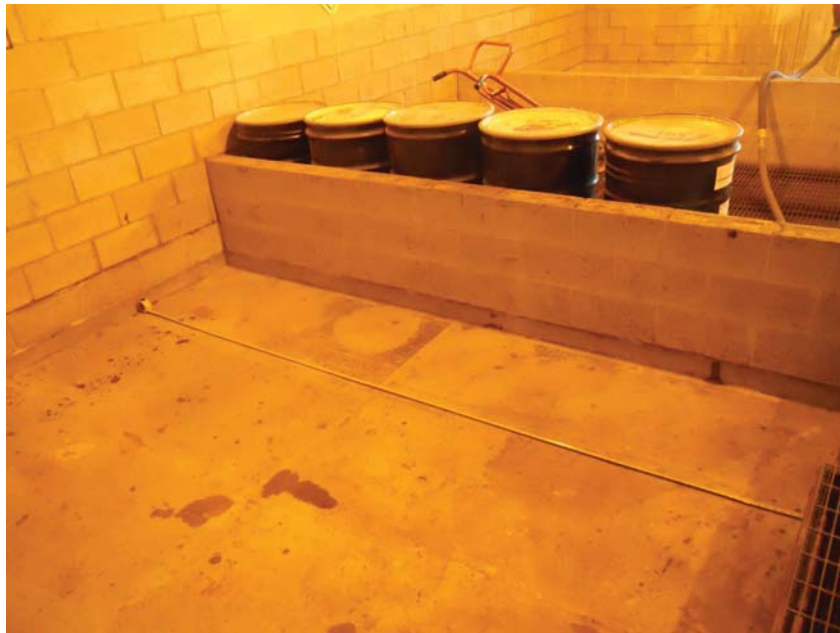
F-2 AND F-3 - NO VISIBLE CRACKS
