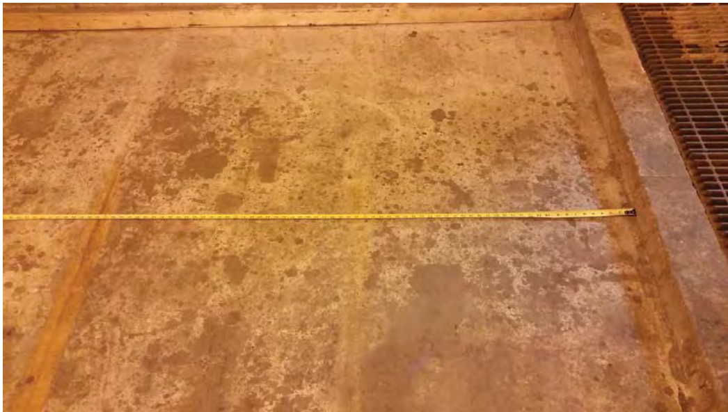
E-5 WEST (1) - NO VISIBLE CRACKS
