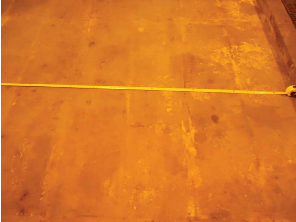
E-2 EAST (3) - NO VISIBLE CRACKS
