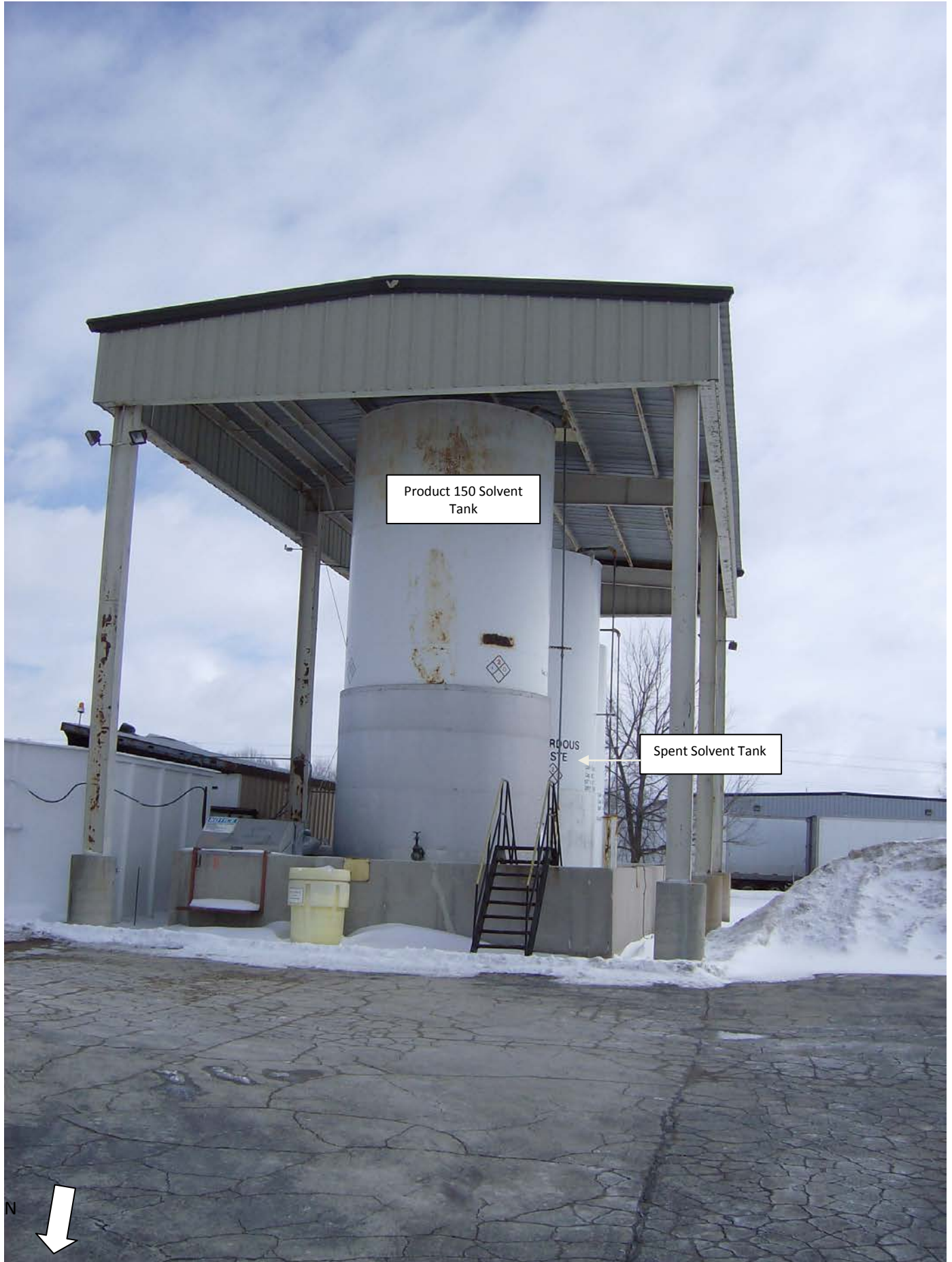
Photo 8. Solvent Tank Farm 2.28.2013
