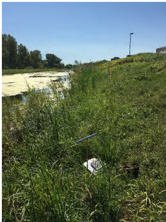
Photo 4. Sample Point P2, view south
