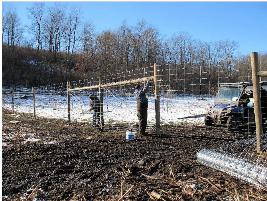
New woven-wire fence being built at Bell Center – December 2016
