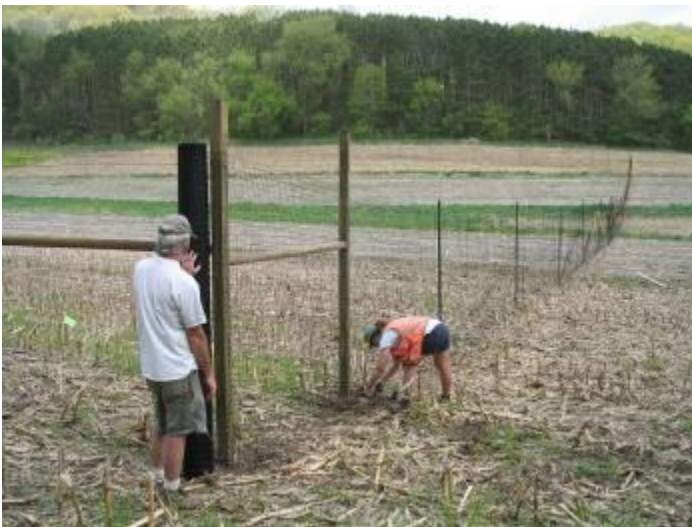
Tree Improvement crew installing deer fence in Crawford County.
