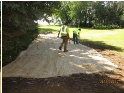
Shoreland gully erosion control project on Fish Lake
