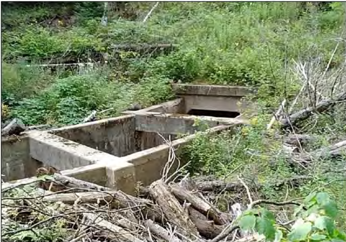
Figure 4. Existing Box Culvert and Channel Side Walls, View Northwest
