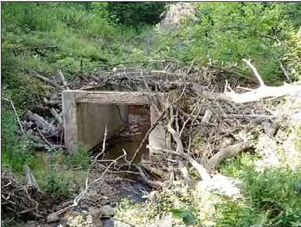
Figure 7. Culvert in Little Balsam Creek South of Trail, View North
