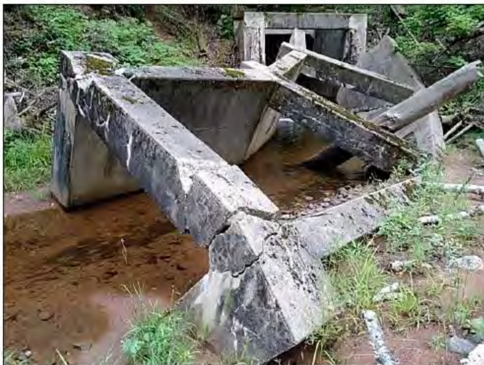
Figure 6. Culvert in Little Balsam Creek North of Trail, View Southwest
