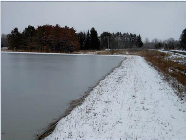
This photo of the infiltration basin in the Flambeau Mine industrial outlot was taken in Spring 2013, when the basin nearly overtopped and had to be pumped (Photo Credit: Wisconsin DNR, April 12, 2013).
