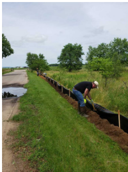
Trench fencing installation. (Nathan Nye)
