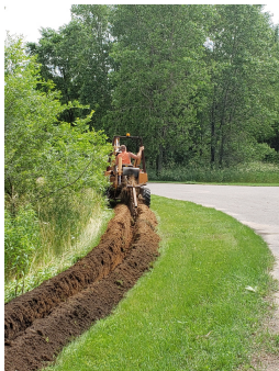
Backfilling a trench. (Nathan Nye)
