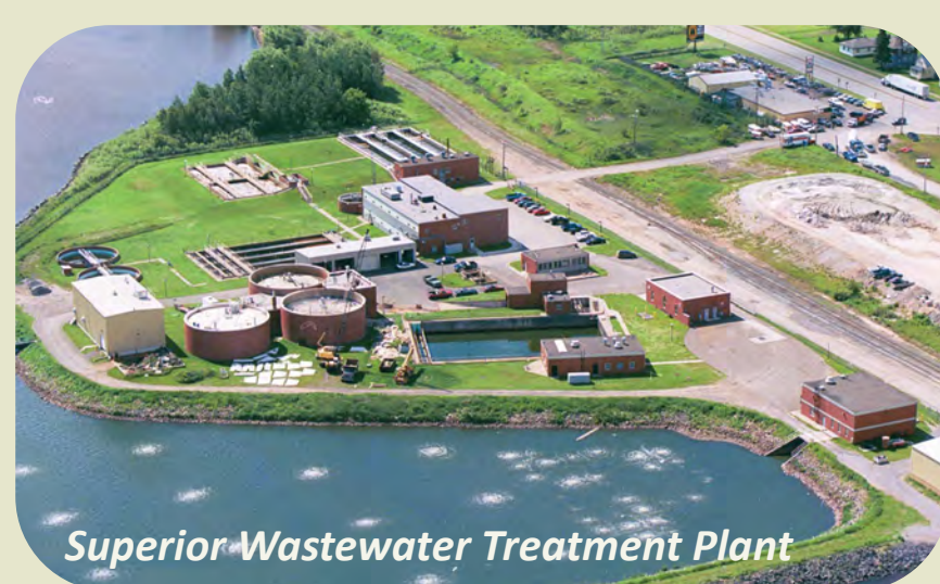
Superior Wastewater Treatment Plant
