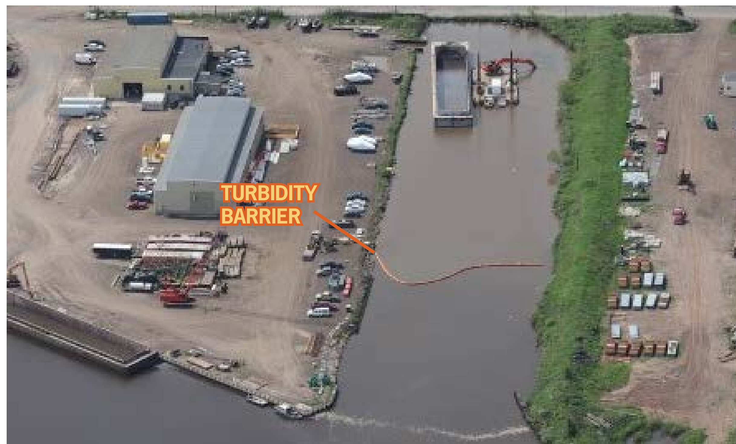
The photo to the left shows a barge dredging sediment in an area protected by a turbidity barrier. A turbidity barrier is an underwater curtain designed to control the spread of sediment from dredging activities.
