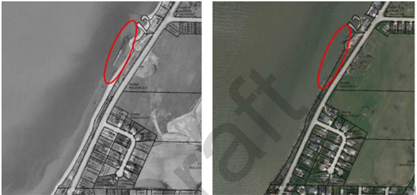
Figure 11. Aerial imagery of Joliet Park and the nearshore area shows the walleye reef shortly after construction (April 2000, 176.14 m monthly average water level – left image) and more recently (May 2020, 177.38 m monthly average water level – right image). The left and right image reflect a change of over 1.2 m/4 ft in water levels. Imagery retrieved from the Brown County “Brown Dog” Geographic Information System (GIS).
