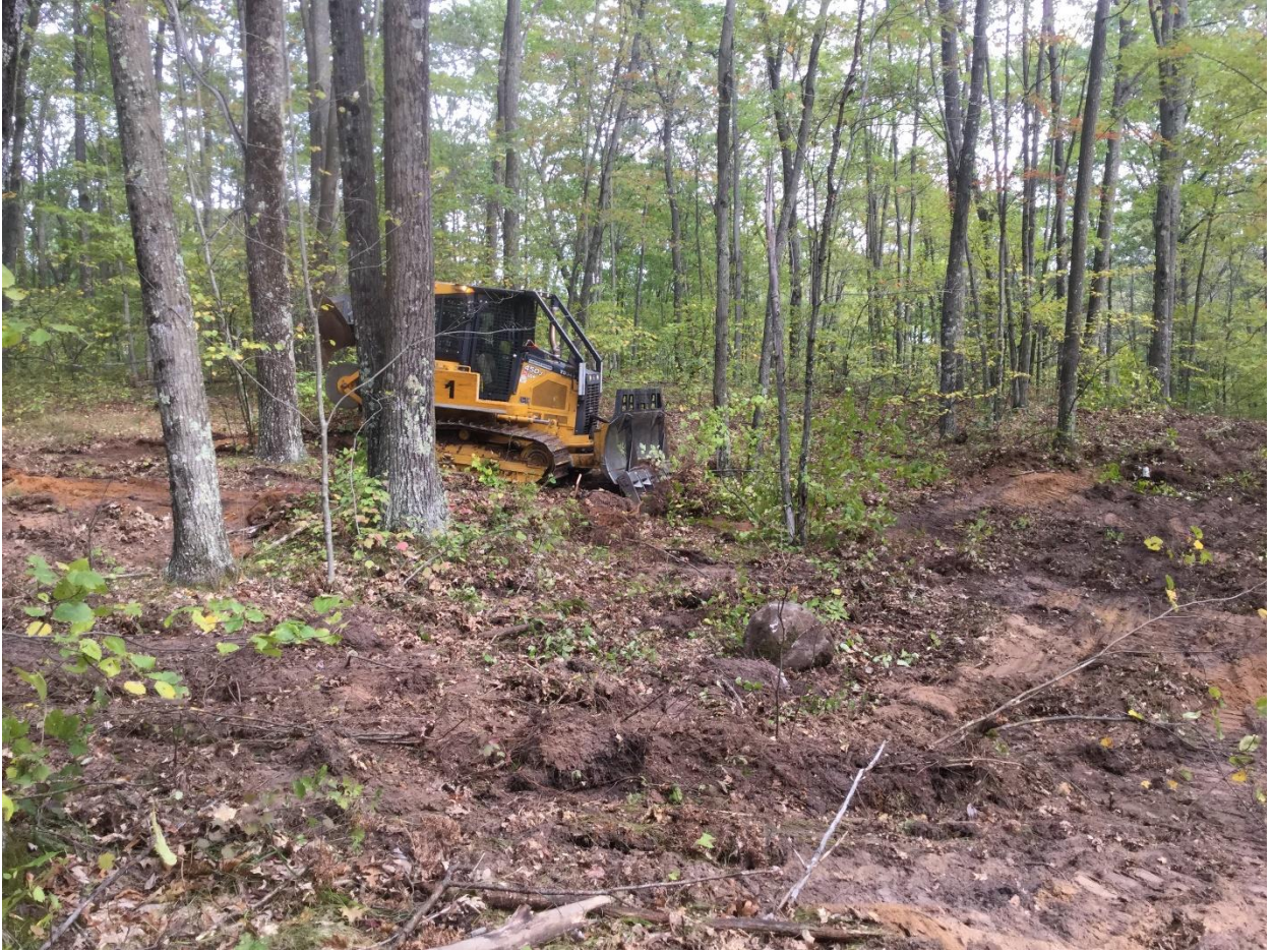
Photo 6 – Salmon blade in operation
