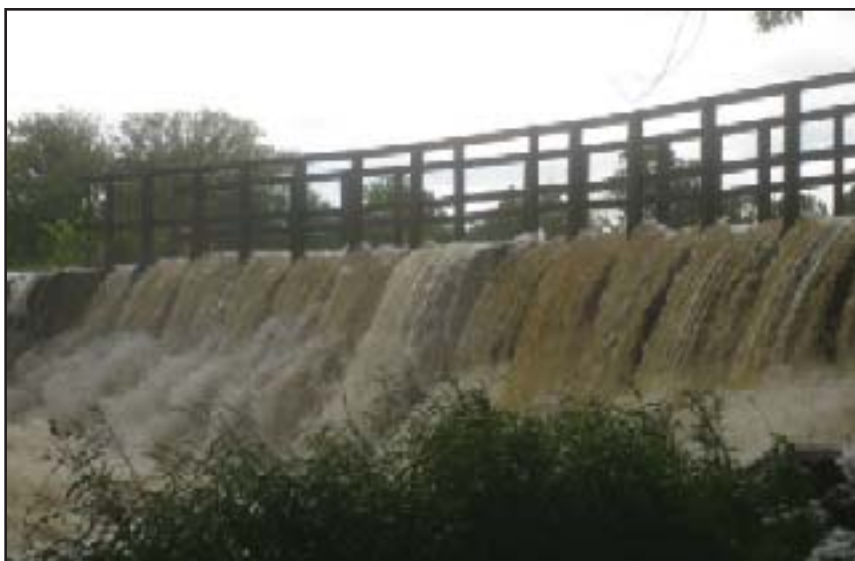
- Overtopping at Saylesville Dam, Waukesha County, June 2008
