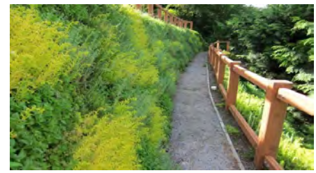
Day 15. Native plant roots grow into and through the soil-filled bags.
