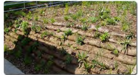
Day 15. Native plant roots grow into and through the soil-filled bags.
