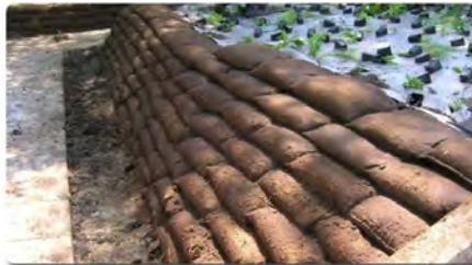
Day 1. Soil-filled geotextile bags are hydro-seeded or planted with native plant plugs.
