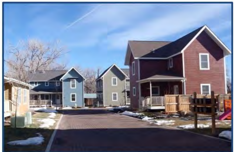
The Toby Lane Development in Boulder, Colorado, remained undamaged in the 2013 flood because the homes were elevated 2 feet above the base flood elevation.
