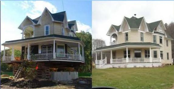
Elevation raises a structure out of the floodplain. Wisconsin has specific regulations to follow with elevation projects. See DNR for more information.
