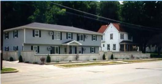
Floodwalls can prevent water from inundating structures that cannot be elevated, relocated, or demolished.
