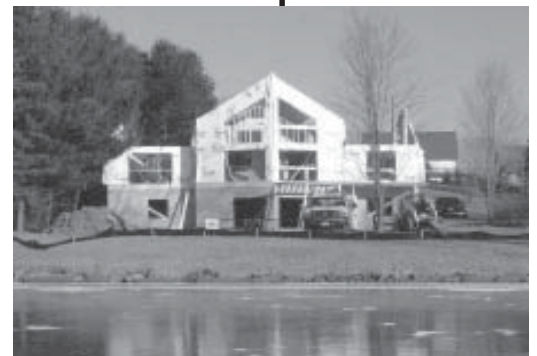
- Shoreline cleared for construction Lake Redstone, WI
