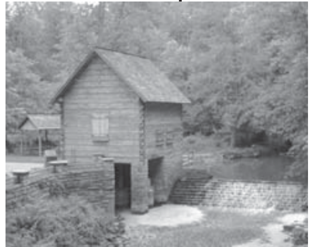
- Mills are just one of the common nonconforming historic structures in Wisconsin
