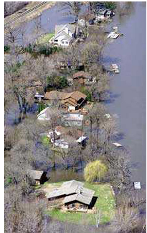
-Elevated homes during flood
