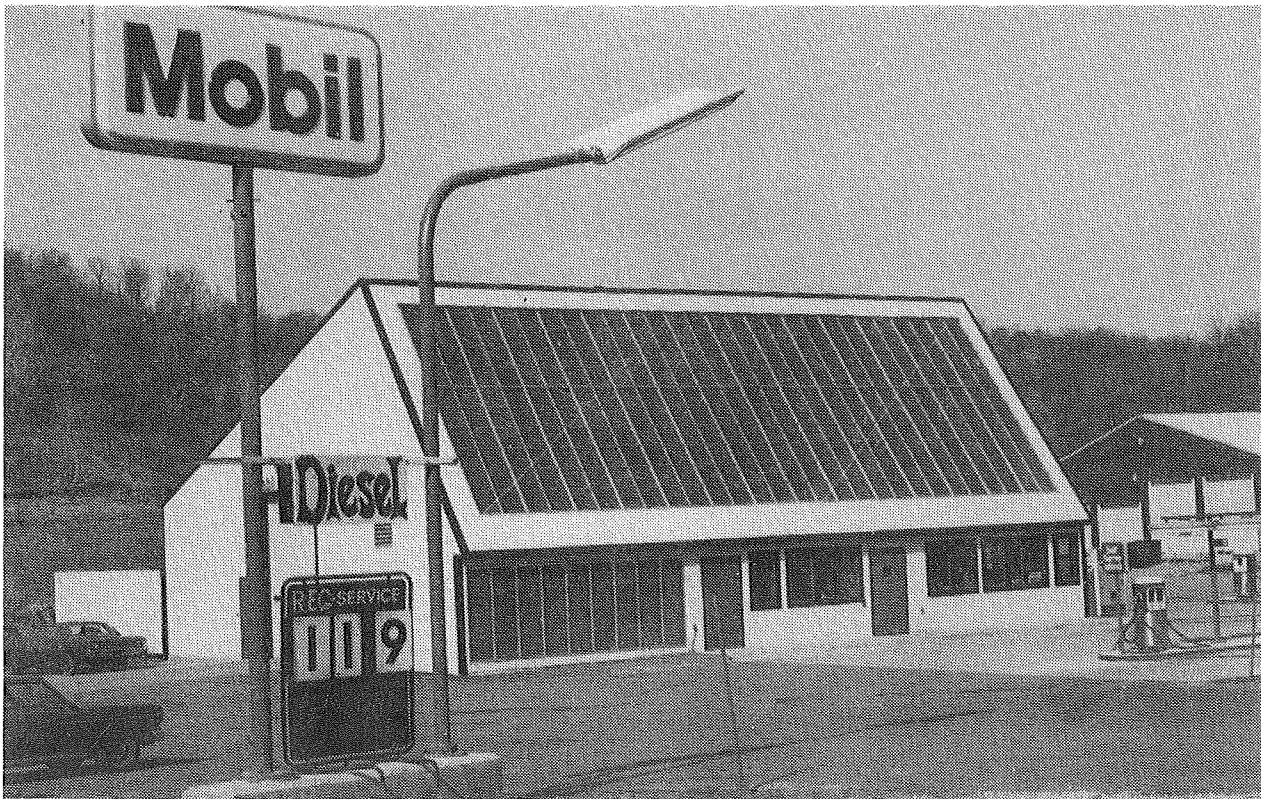
Even in Wisconsin's northern climate, solar heating systems can provide an average of 75 percent of each building's heating needs, when the simple, site-built systems are combined with high levels of insulation and intelligent building design.
