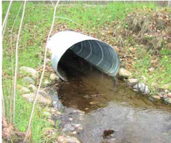
Beneficial culvert placement.
