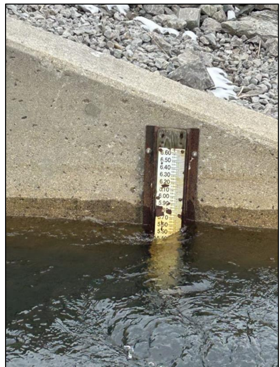
Image 4: Stationary gauge located on the upstream side of the Eldorado Marsh Dam. Photo Credit: Wisconsin DNR.
