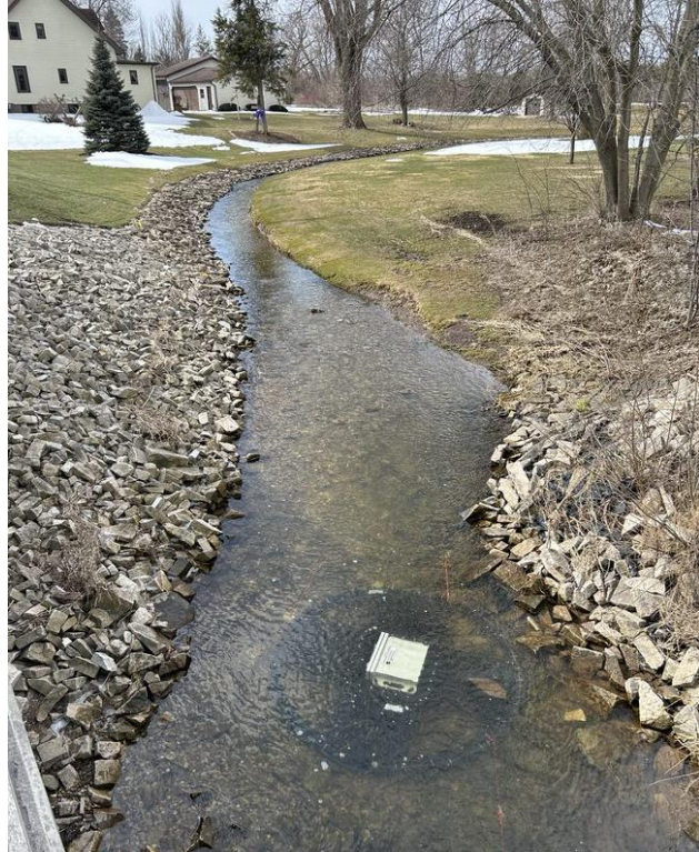
Image 3: Submersible disc array located at Van Dyne Road. Photo credit: Wisconsin DNR.
