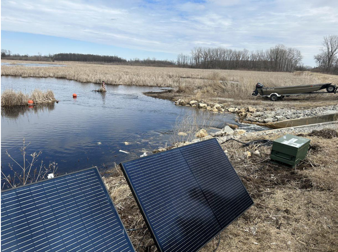
Image 1: LITZ cord solar set up located at the Eldorado Marsh Dam. Photo credit: Wisconsin DNR
