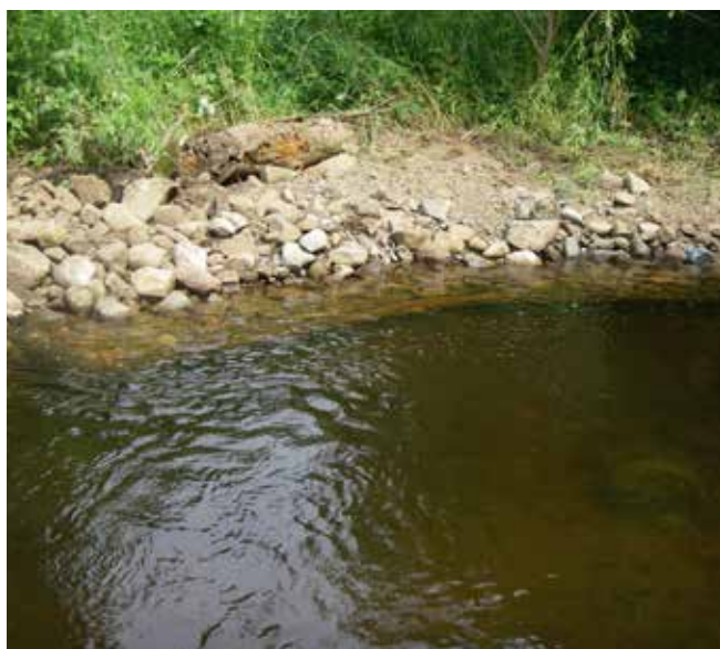
LUNKER structure deployment on the North Fork Clam River, Burnett County.
