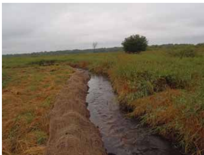
The Scuppernong River project restored a stretch of river to its original channel. Biologs and erosion control mats are used to stabilize the new stream banks.
