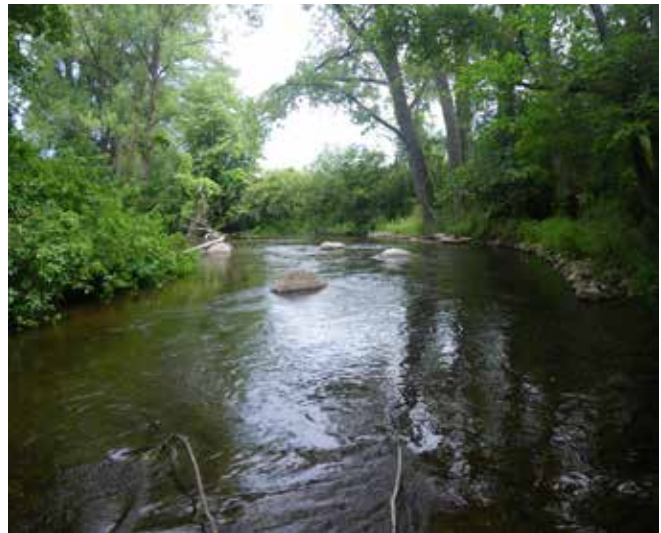
Lunker boulder installation Tomorrow River, Keener Road, Portage County
