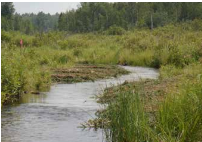
The installation of brush bundles on Mary Creek, Oconto County.
