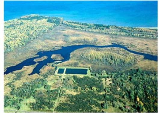
Port Wing wastewater lagoon restoration site
