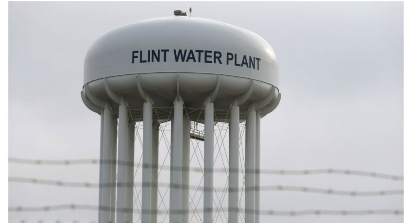
The top of the Flint Water Plant tower is seen in 2016 in Michigan. Rebecca Cook/Reuters
