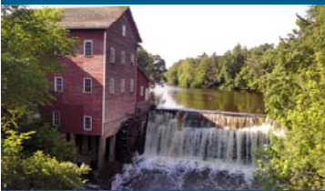
Dells Lake Dam
