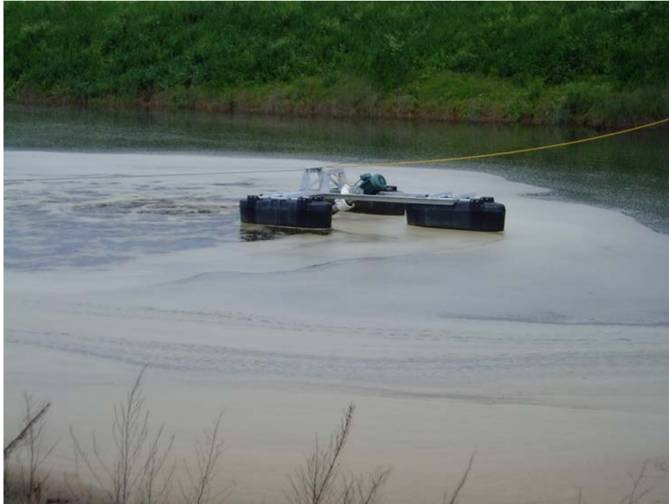
Figure 4.2 Floating Aerator on Secondary Basin
