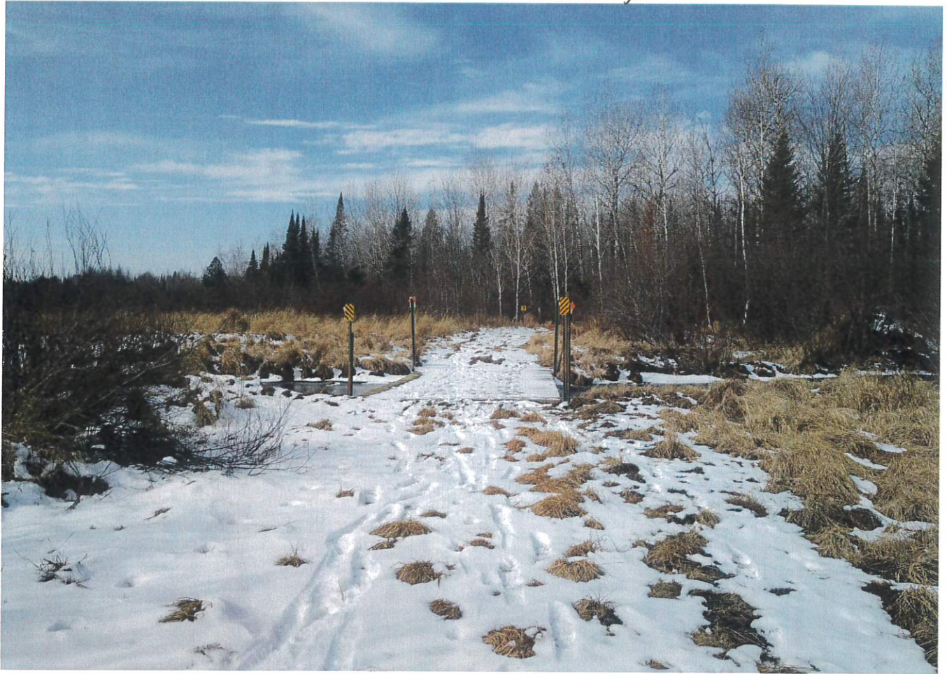
Dear Creek Snowmobile Bridge
