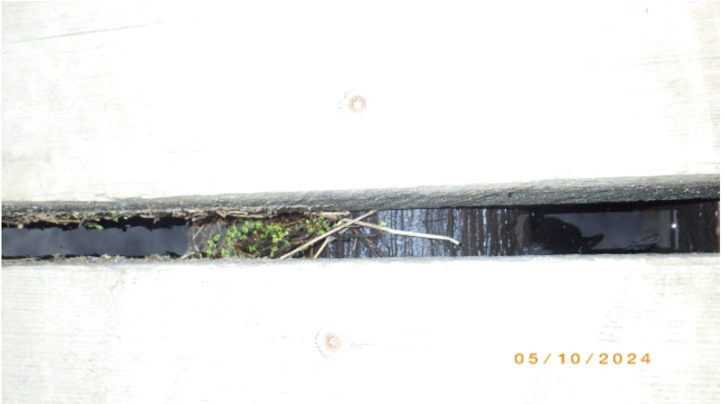
Very decayed timber superstructure.
